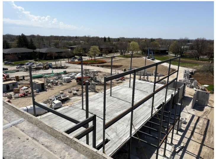
Aerial View of Structural Steel & Precast- Area C
