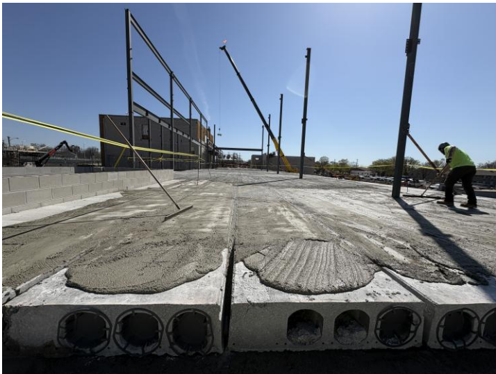
Precast Grouting Level 1 - Area C
