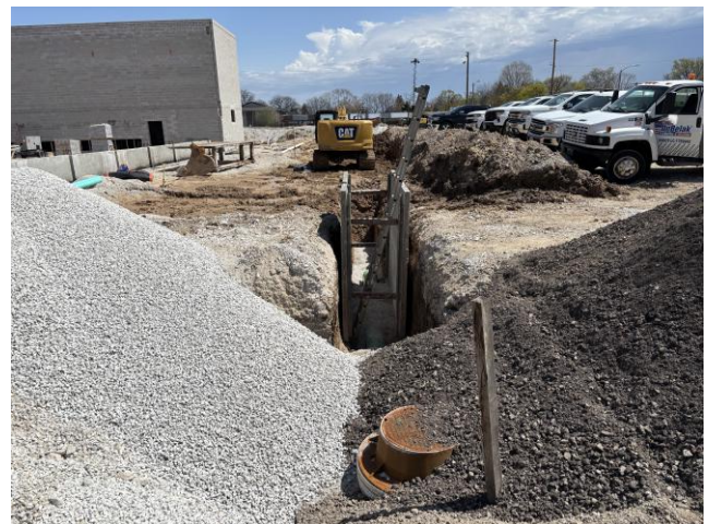
Storm Structure Installation– South Parking Area
