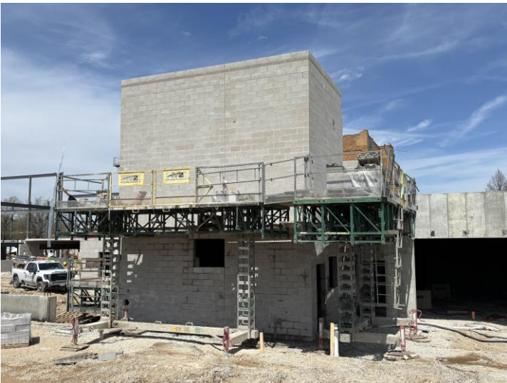
Exterior CMU Walls- Storage & Fire Pump Rooms Area B
