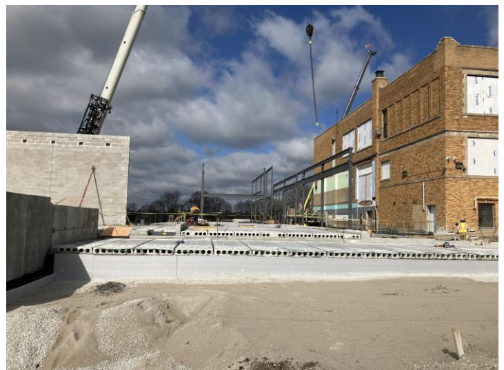
East Foundation Backfill Following Precast Erection- Area B
