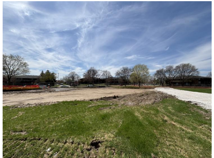
Playfield Site Grading & Stone Access Roads- Pump Track
