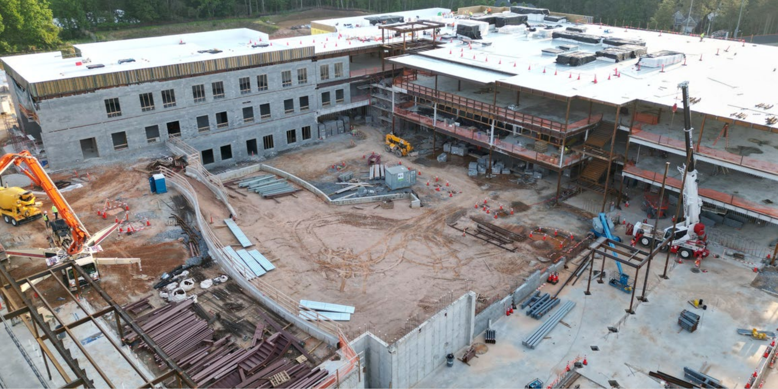
Area '2' and '3'- External Masonry
