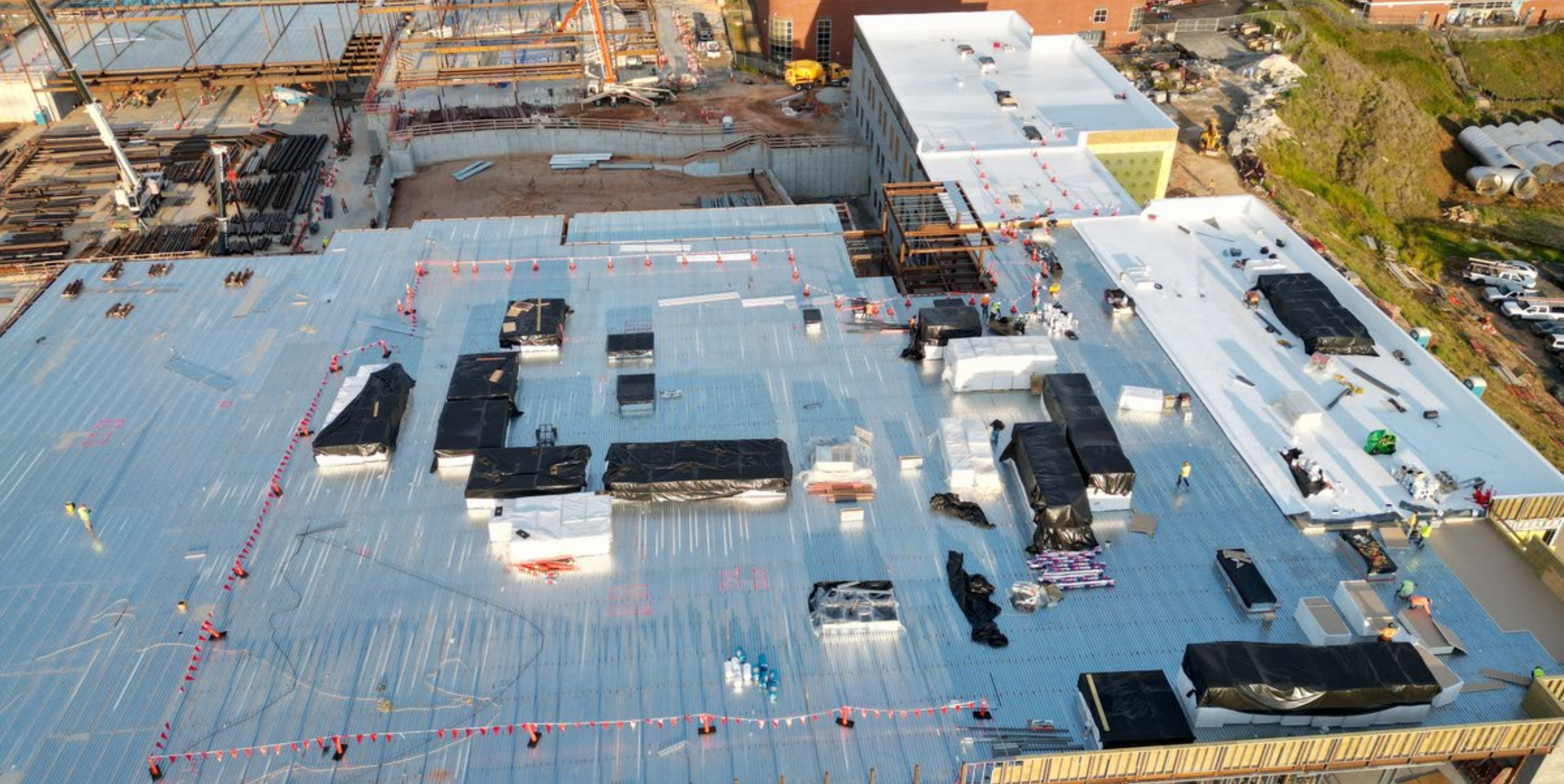
Area '4' Roof in Progress.
