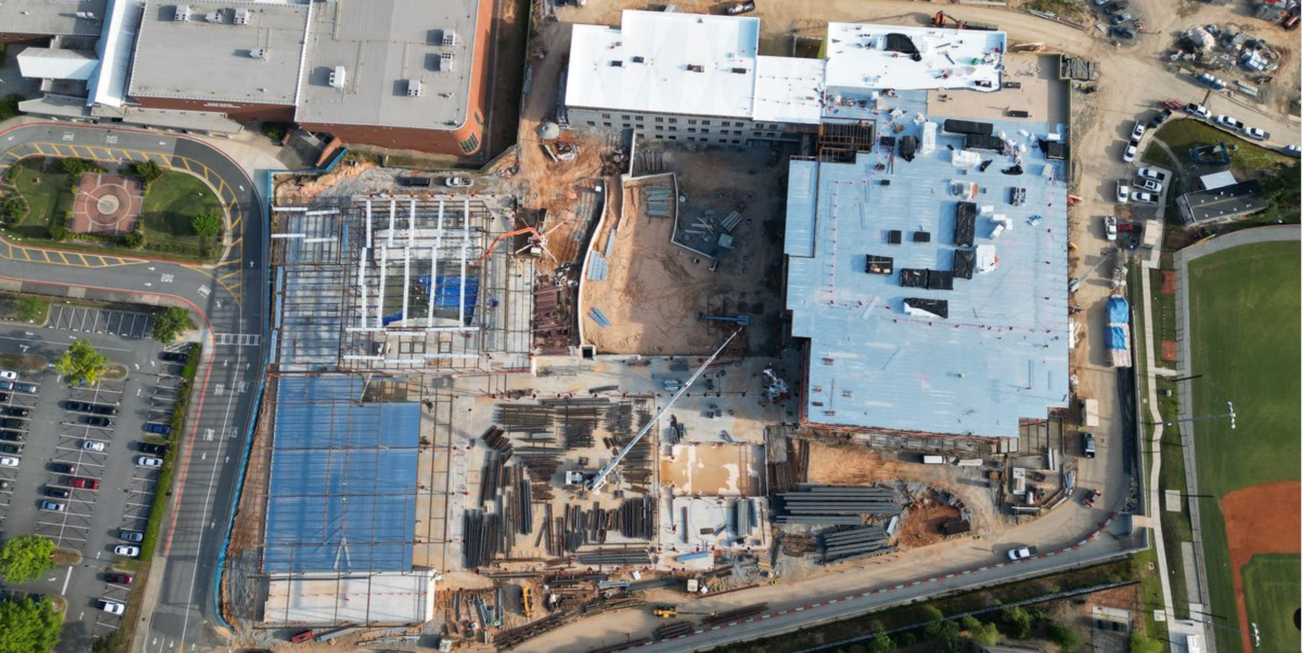
Overall Site Progress
