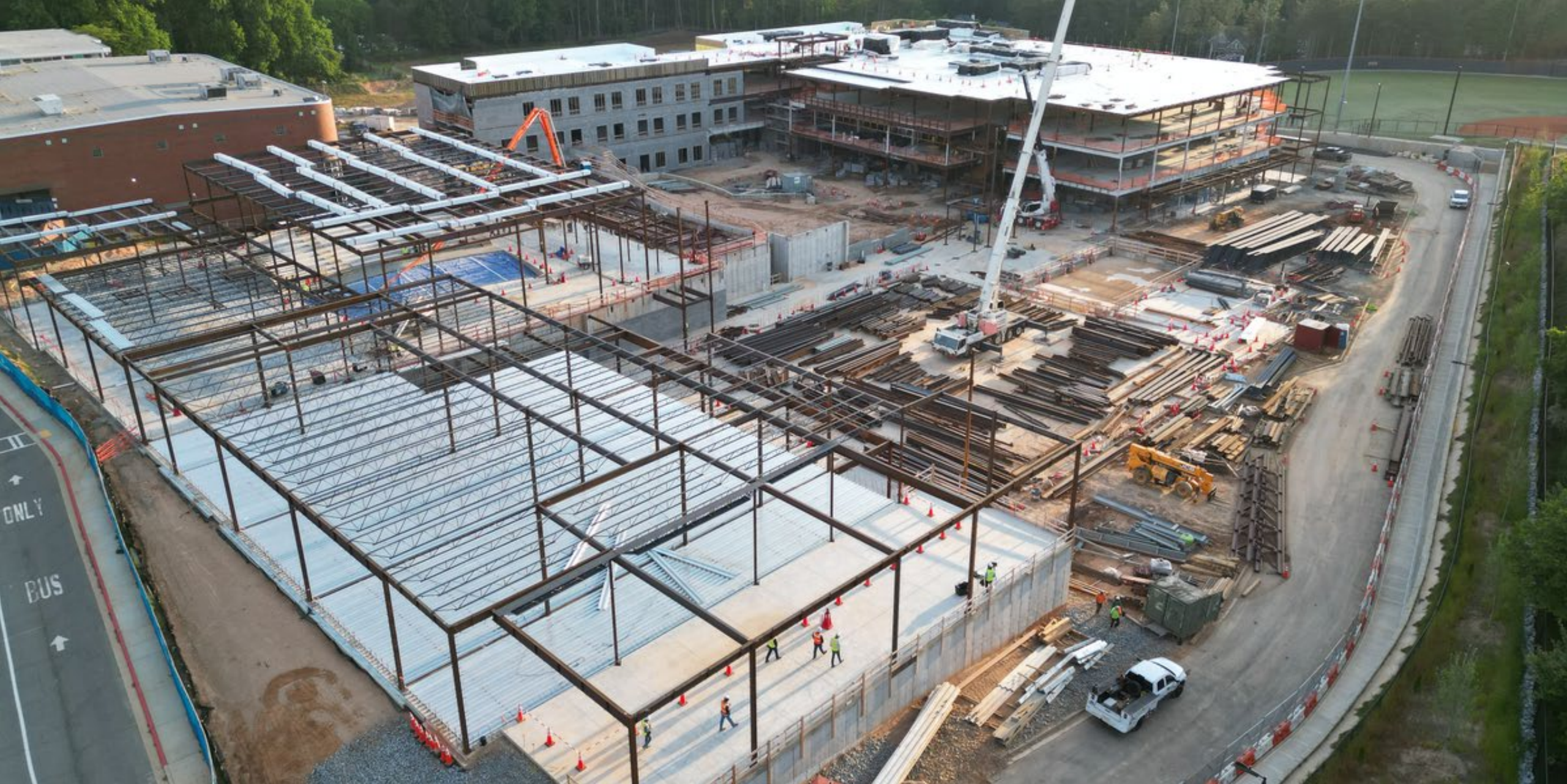
Area 7- Gymnasium and Area 8 Auditorium- Steel Erection
