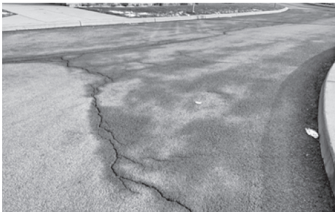
Existing parking lot
