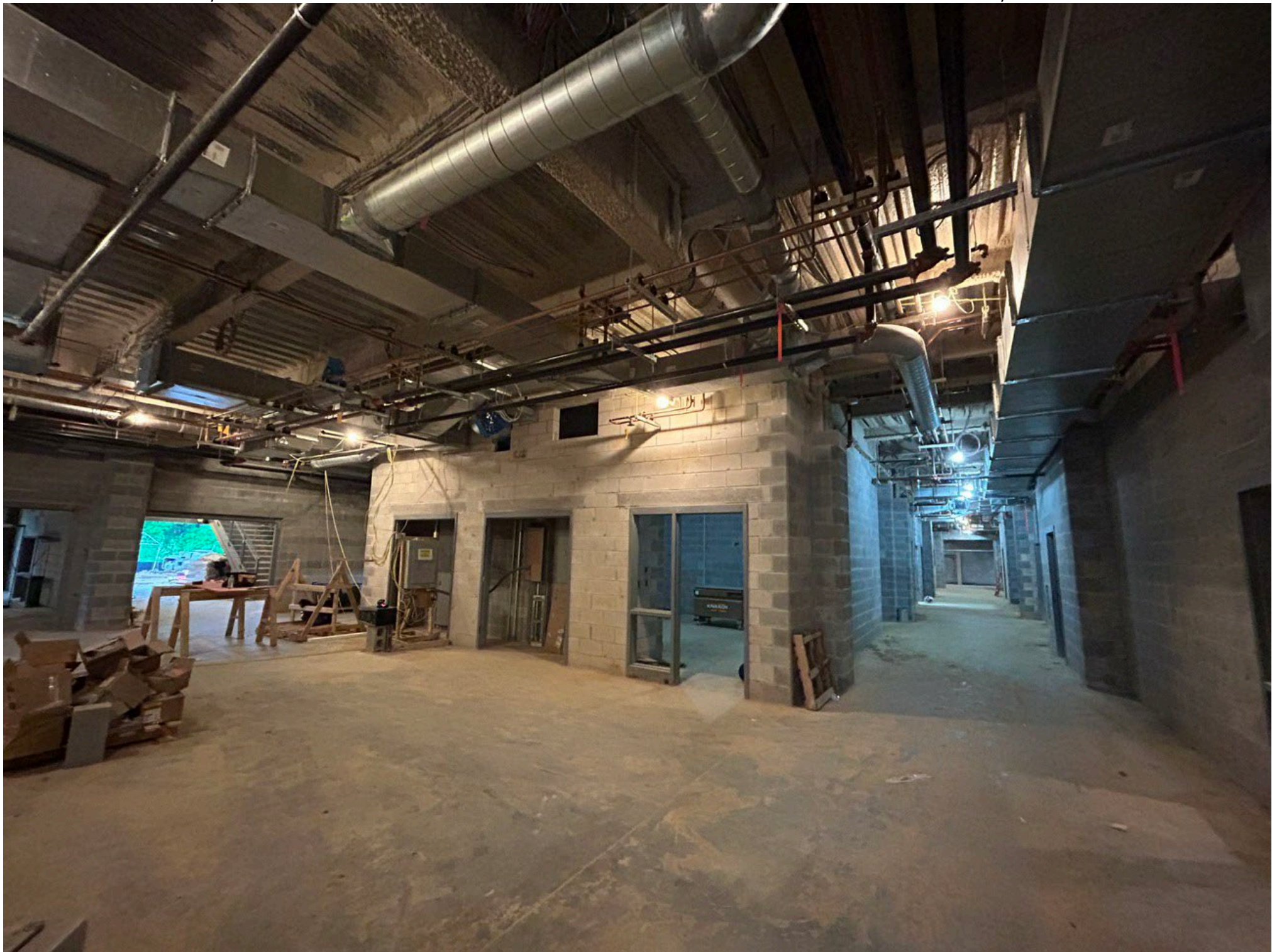
NORTH EAST MIDDLE / HIGH SCHOOL – REPLACEMENT – AREA C – MIDDLE SCHOOL WING COLLAB AREA / CORRIDOR
