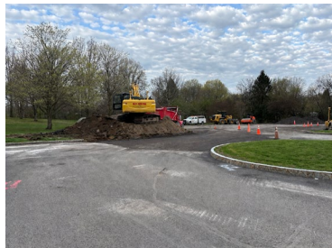
HS Parking Lot
