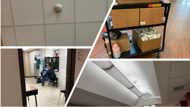
Smoke Detector Replacement
