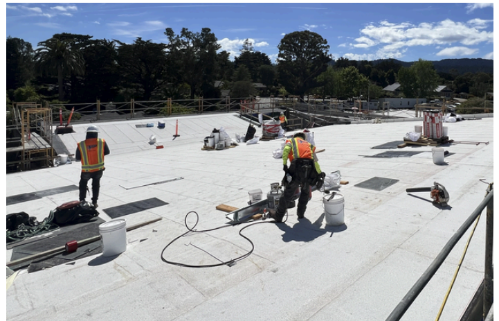
PICTURED ABOVE: Roofing contractors working on waterproofing the MPR.
