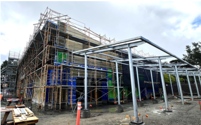
PICTURED ABOVE: Canopy structures are up!
