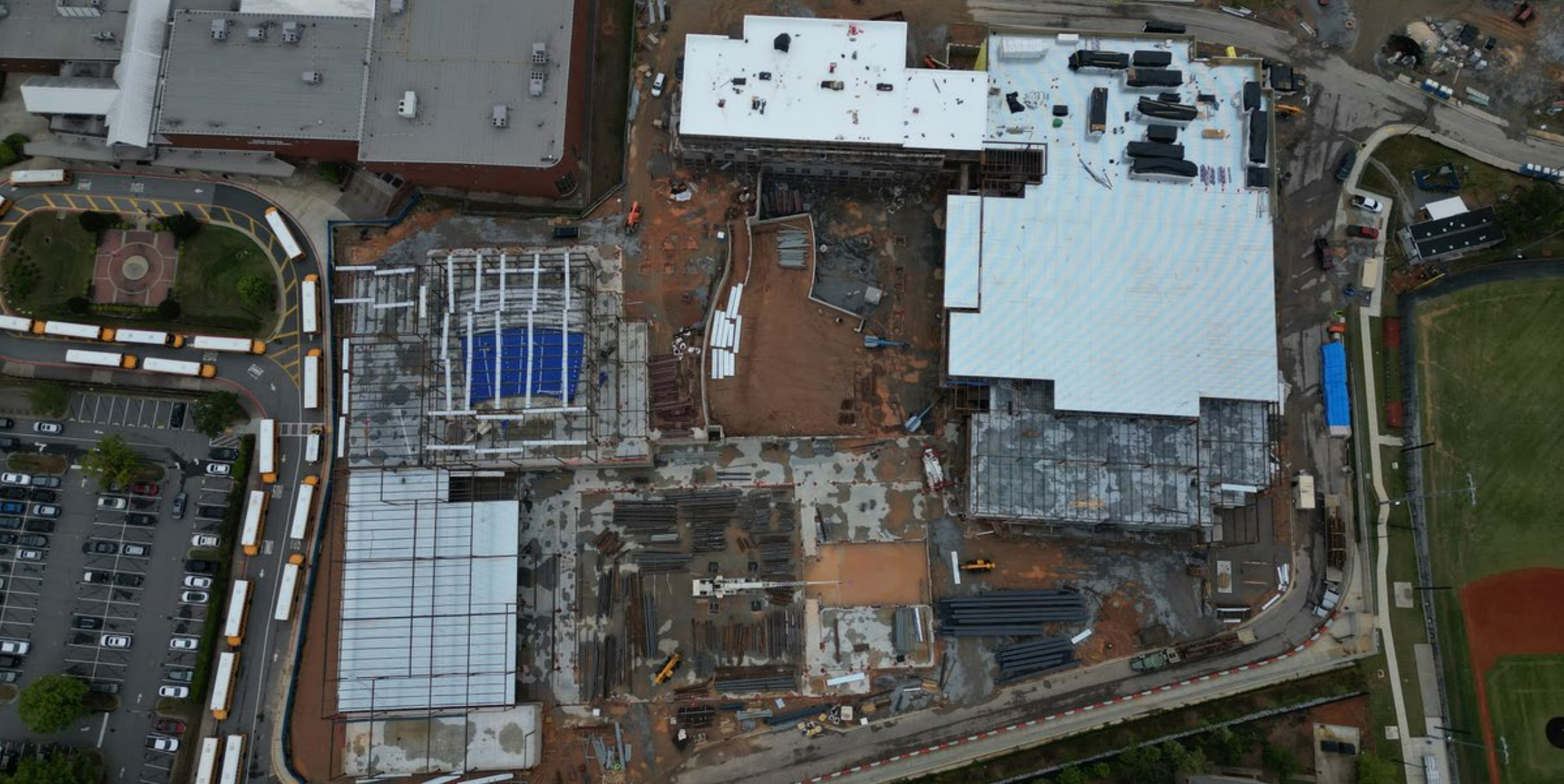
Overall Site Progress- 2
