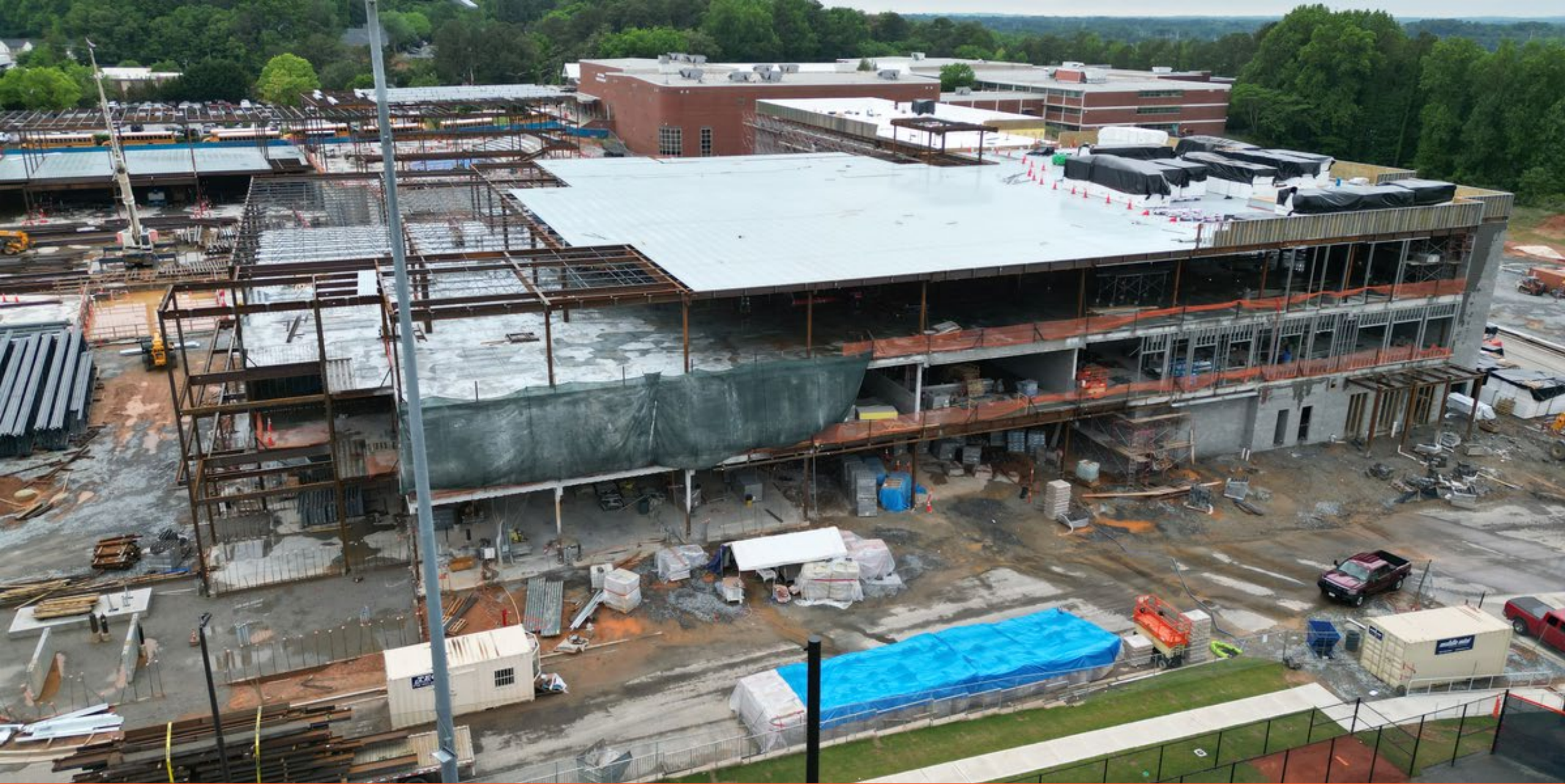
West Elevation- External Framing and Roof work.
