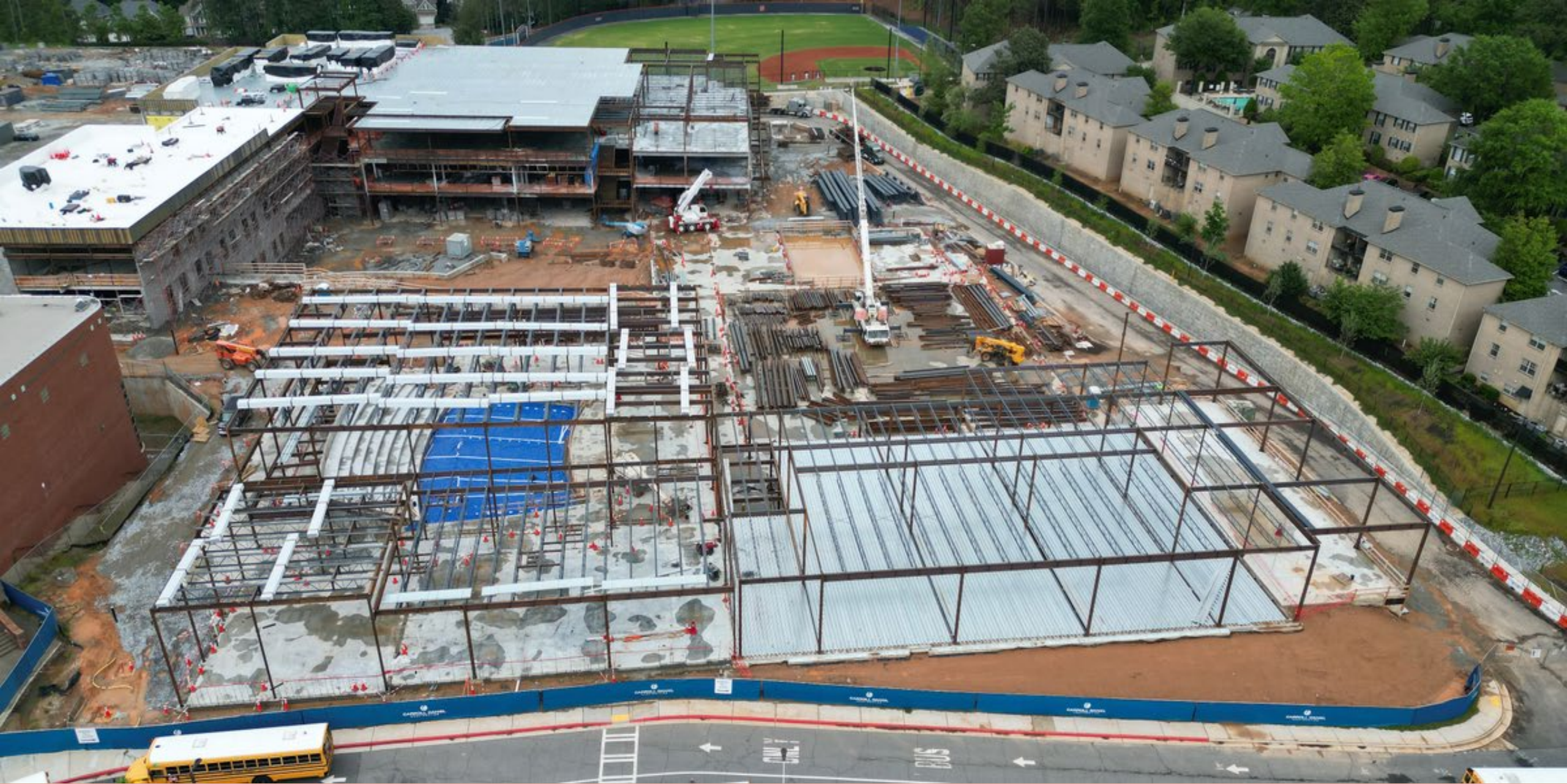
Area 7- Gymnasium and Area 8 Auditorium- Steel Erection
