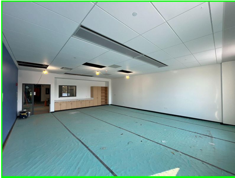
Classroom progress: cabinetry and millwork installation underway
