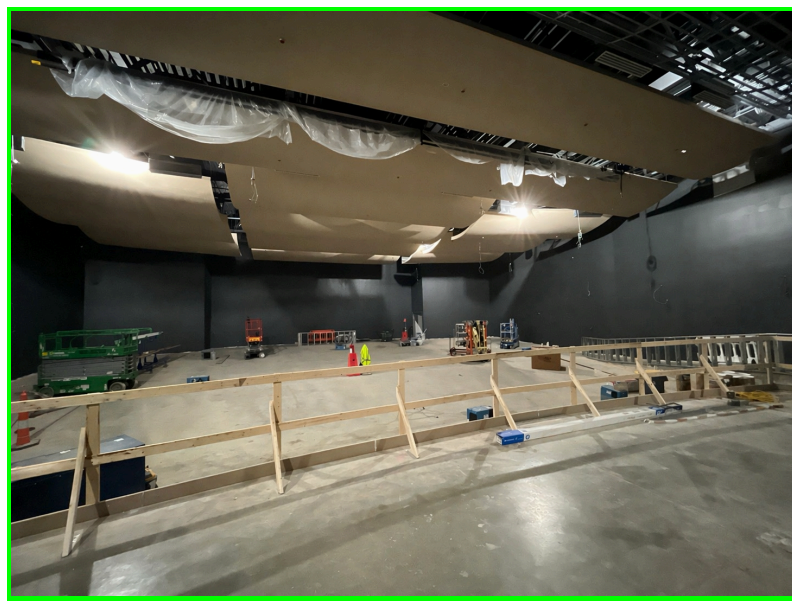
Auditorium progress: view from the stage toward the future seating area, with acoustic clouds installed above to manage sound
