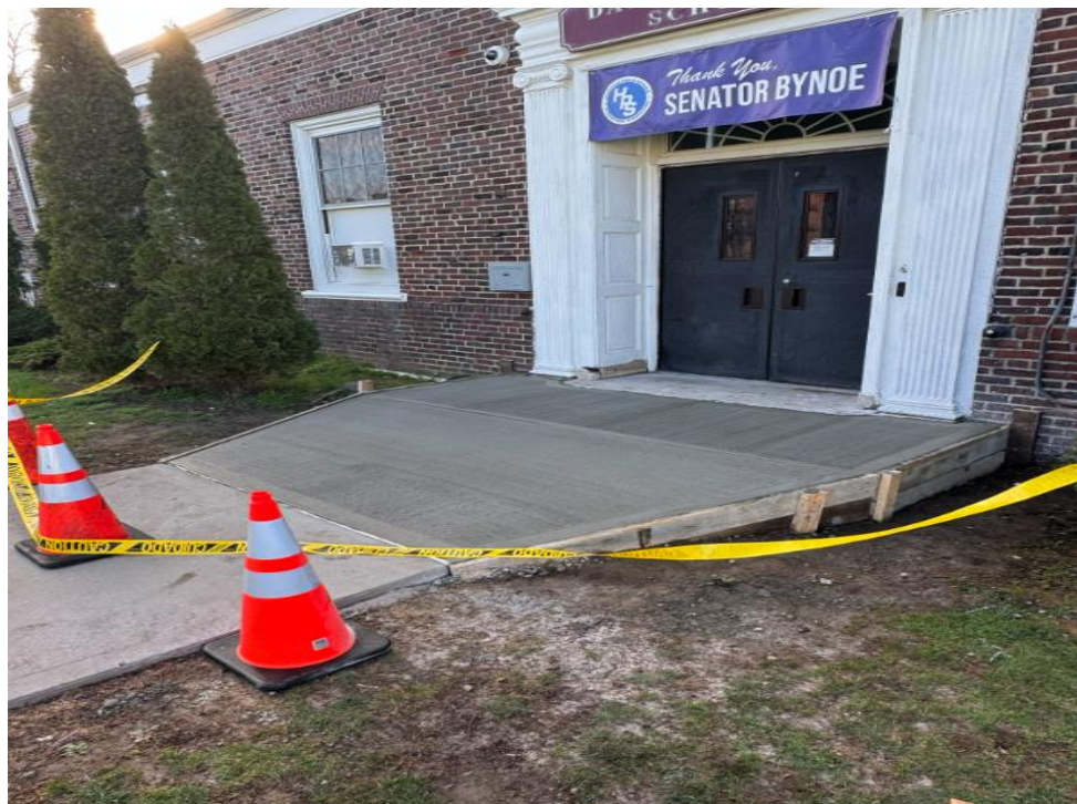
Hempstead 2022 Bond Ph. 3 – Concrete Work
