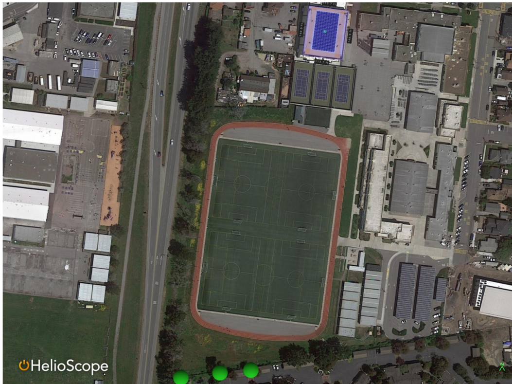
Cunha Intermediate School – Event Center Roof Top Array
