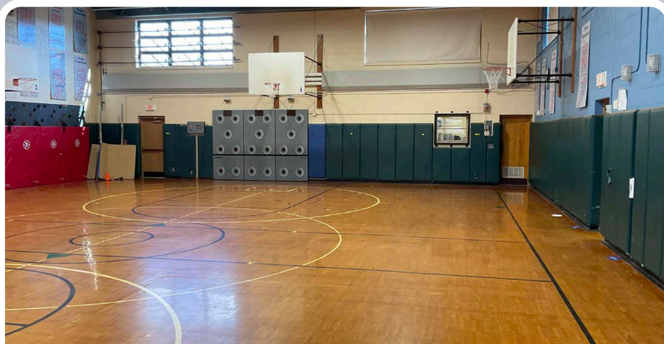
EXISTING GYM WALL PADS/ BACKBOARDS
