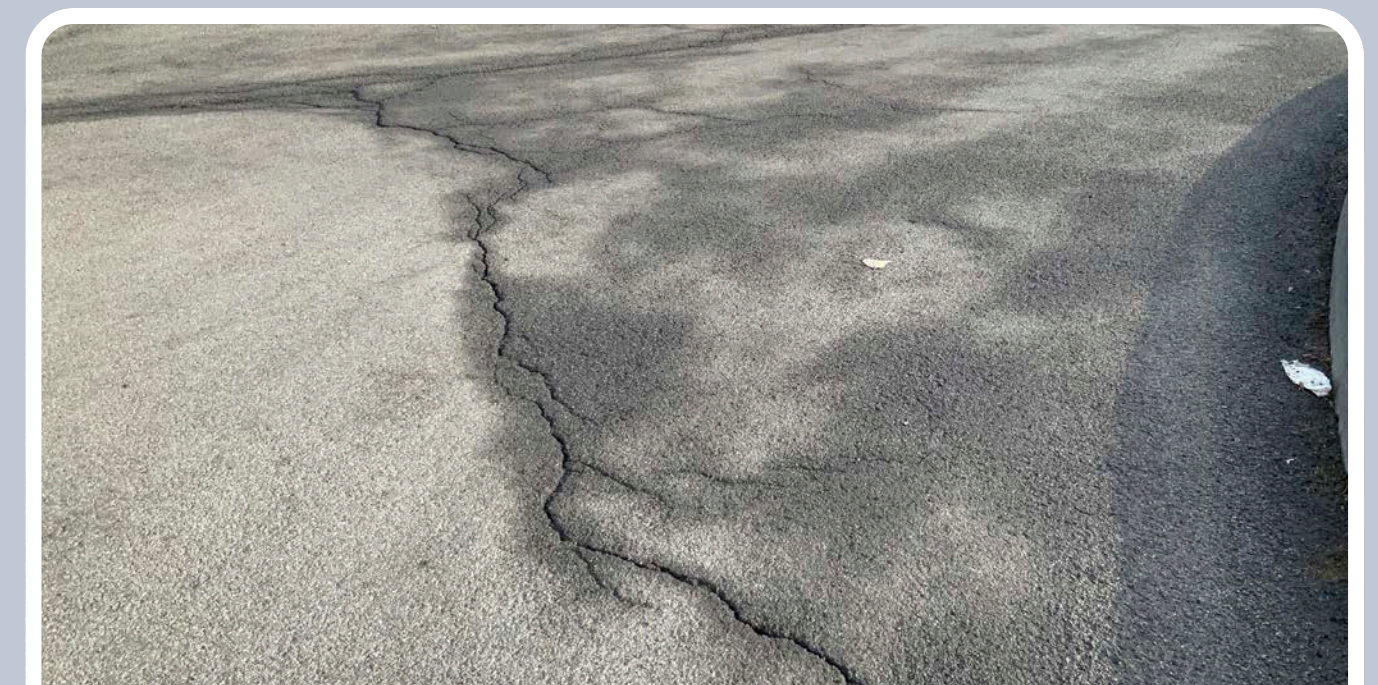
EXISTING PARKING LOT
