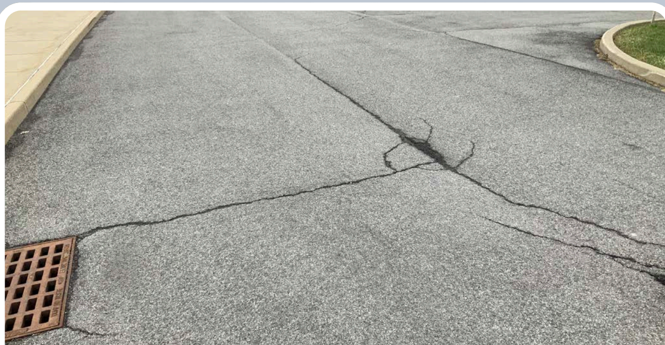
EXISTING PARKING LOT
