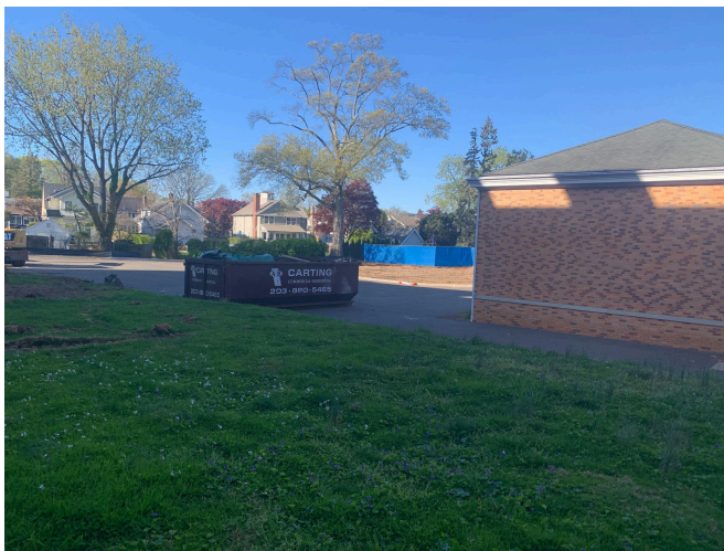
Old playground demolished, site prep underway
