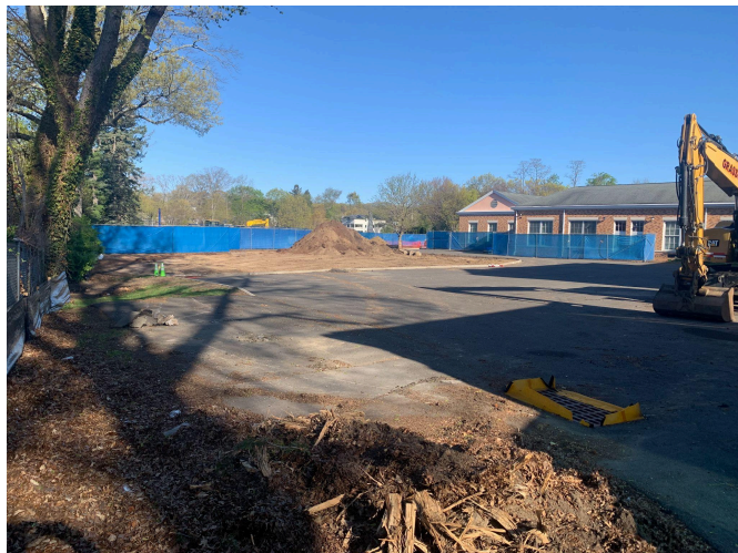
Construction fencing, erosion control measures in place
