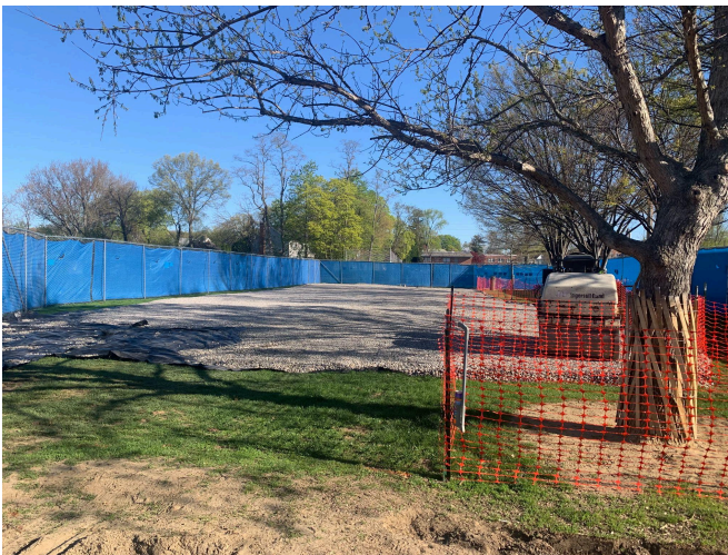
Tree protection installed, staging/storage area developed
