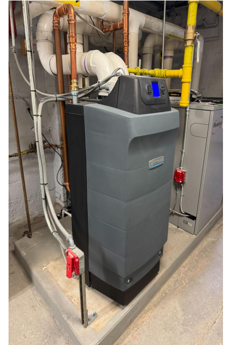
Boiler Replacement at Watchung
