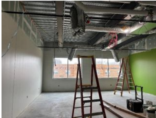
Area B Classroom Paint
