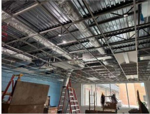
Area F Classroom Ceiling Grid
