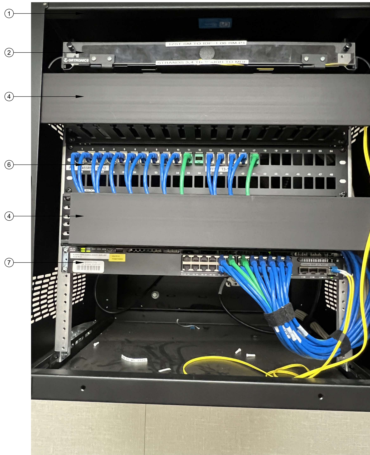
RACK - EXISTING CONDITION
