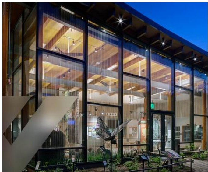
4B- Main Expanses of Glass (Curtainwall) @ front of School Cafeteria, Media Center & Gymnasium
