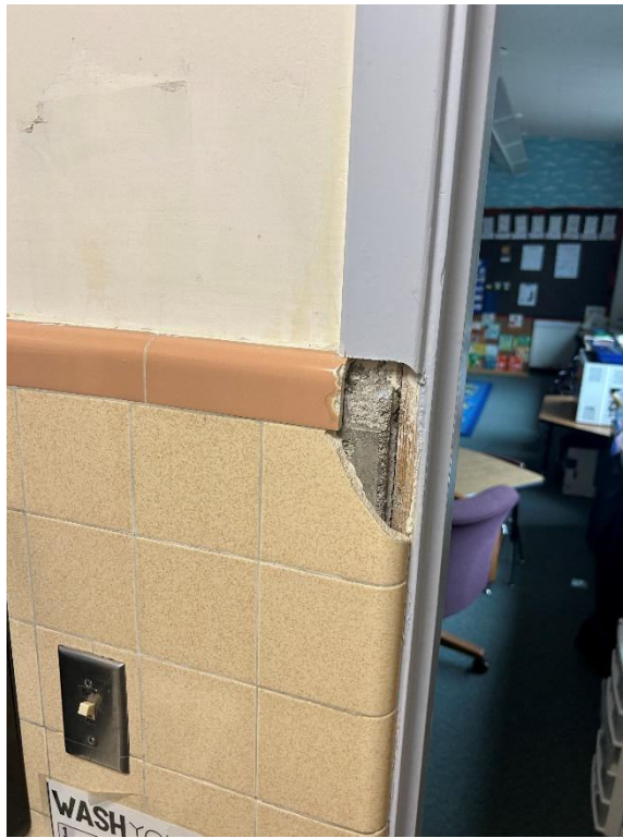
Concrete and grout sampling location
