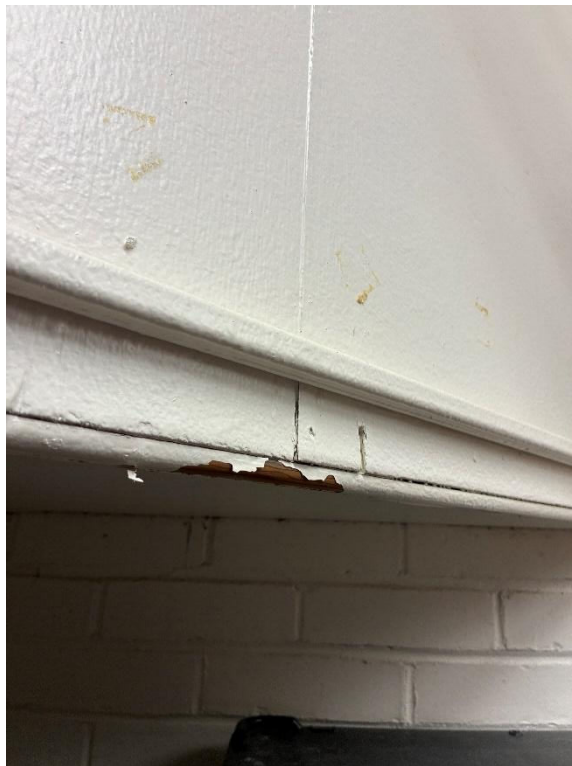
Paint sampling location – negative for lead based paint coatings
