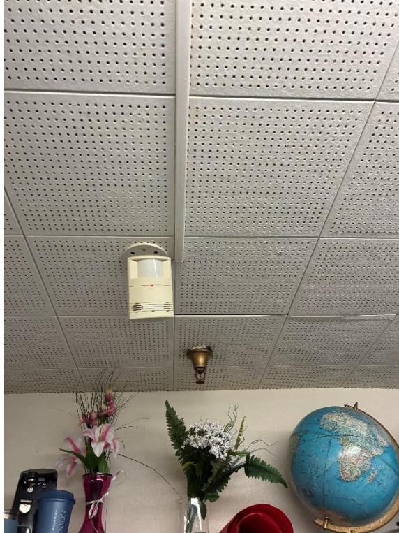
Ceiling tiles through out – negative for asbestos
