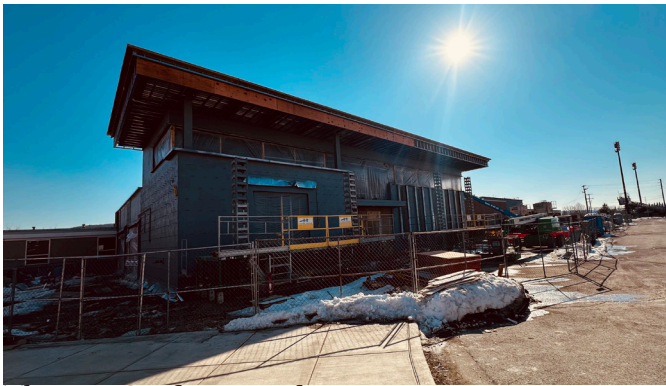
The PVHS cafeteria mid-renovation
