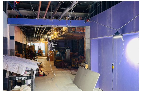
An empty PVHS hallway under construction
