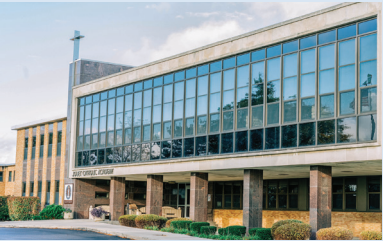
“Honoring Our Past” Windows and Air Conditioning Wi-Fi Infrastructure
