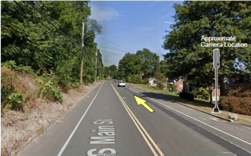
S. Main St (Looking North)
