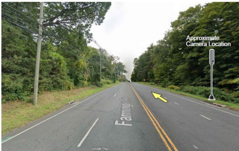
Farmington Ave (Looking West)
