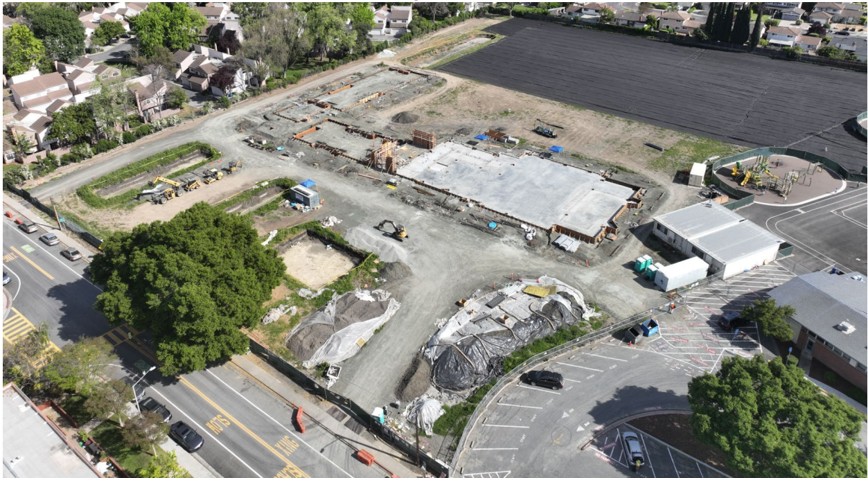
Aerial view looking northwest on March 25, 2026.
