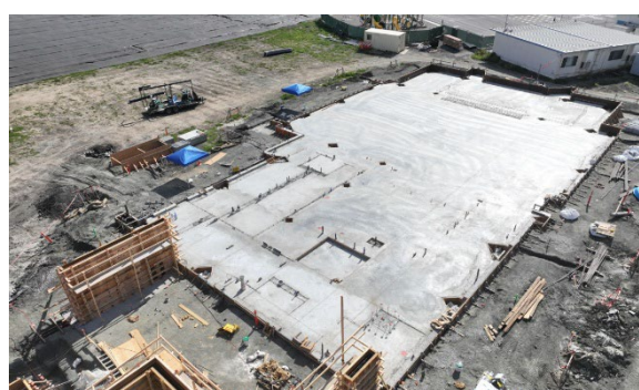
Multipurpose Building Floor Slab
