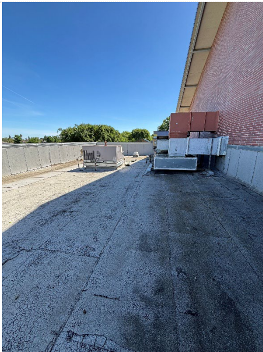
Cafeteria South Roof
