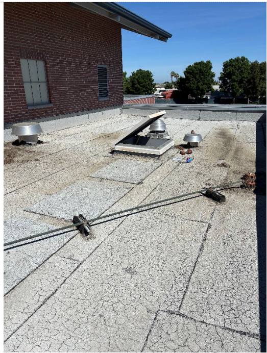
Cafeteria North Roof
