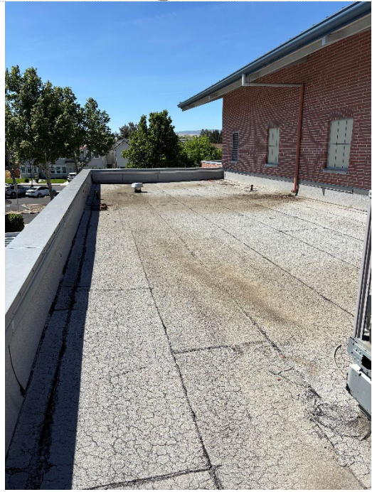
Cafeteria East Roof
