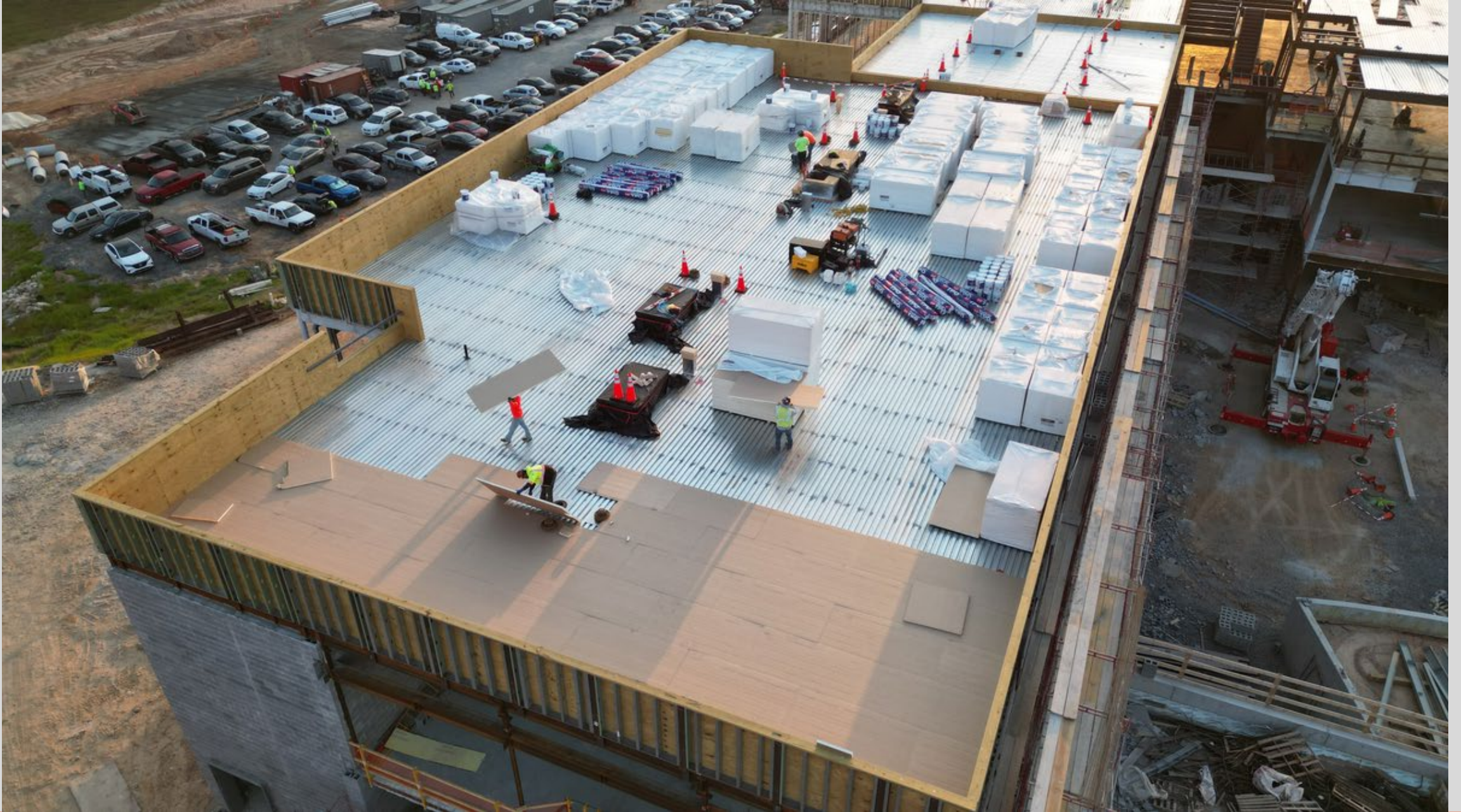
Area 2 and 3- Roof
