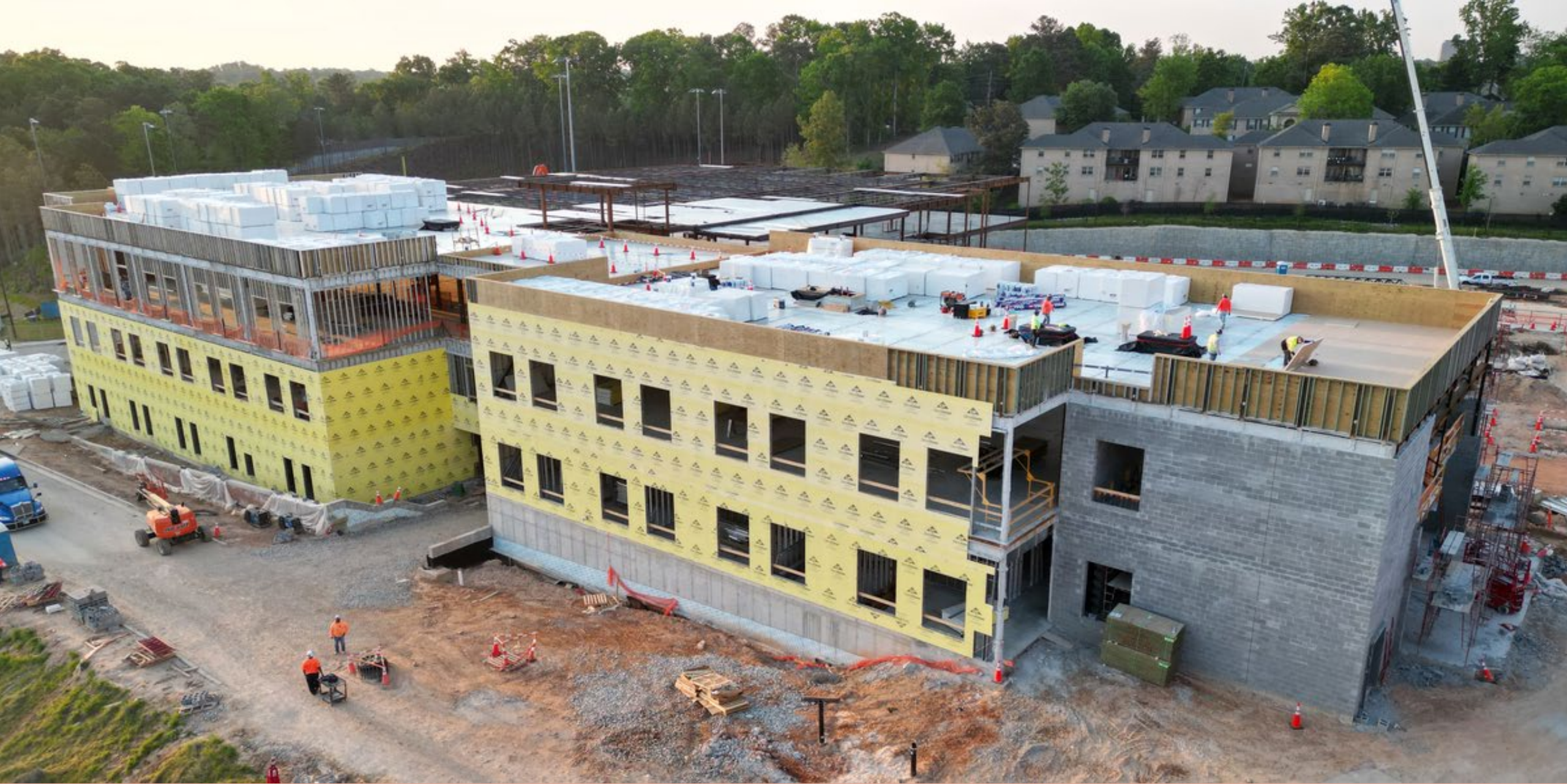
External framing and masonry
