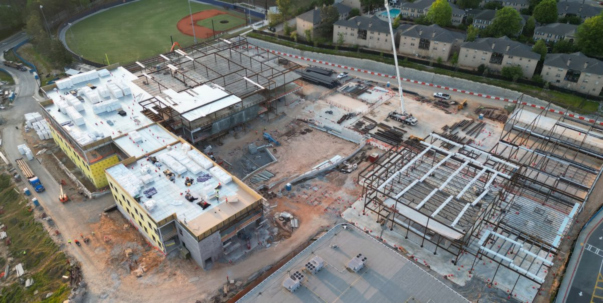
Overall Site Progress
