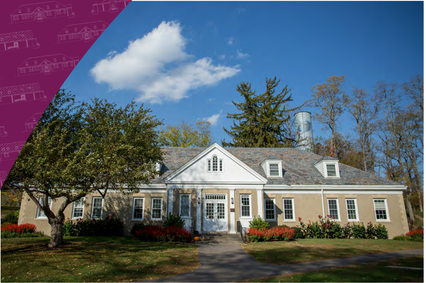
When first-floor renovations are complete, Hoffman House will have an additional 15 beds for boarding students.
