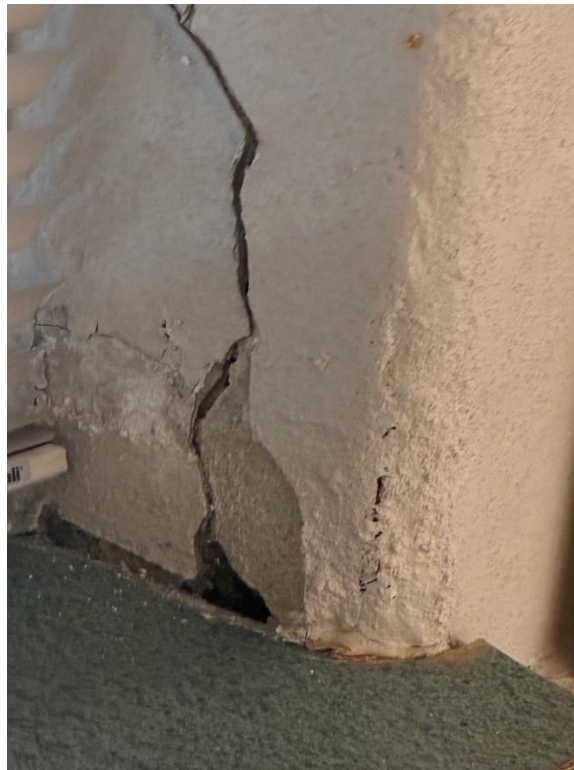
Plaster cracks
