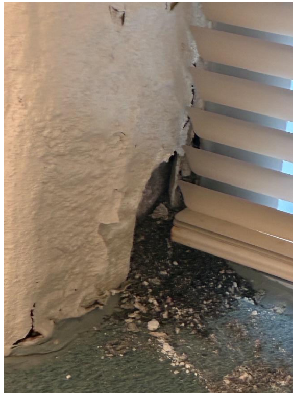
Corrosion evidence from steel beam
