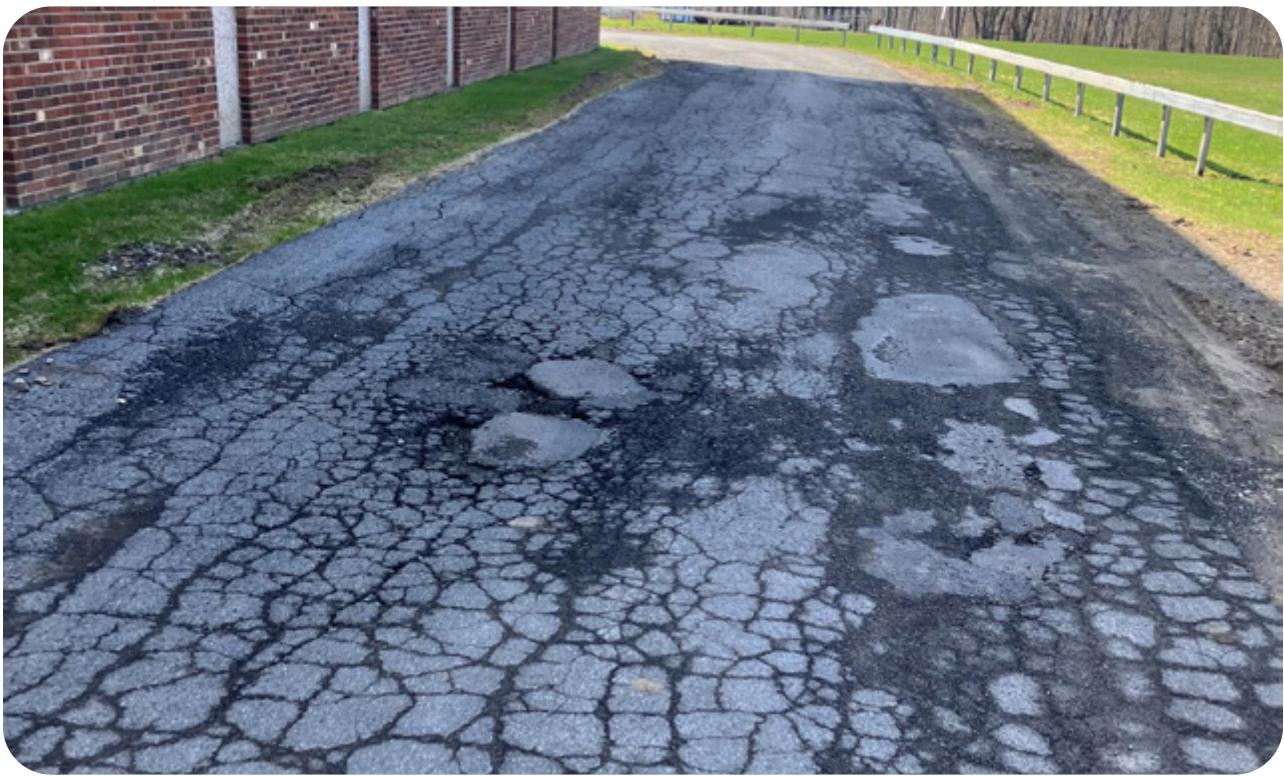
Deteriorated pavement
