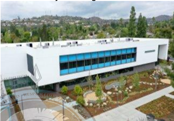
New Two-Story STEM Classroom Building
