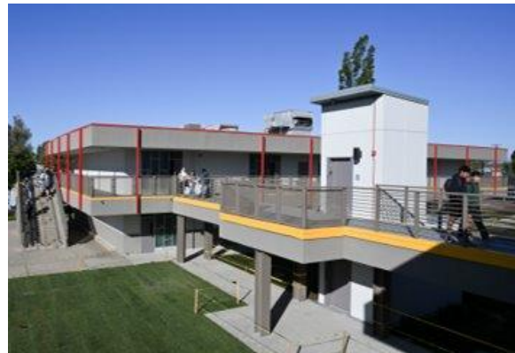
Modernized Classroom and New Furniture
