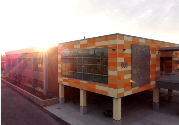
New Two-Story STEM Classroom Building
