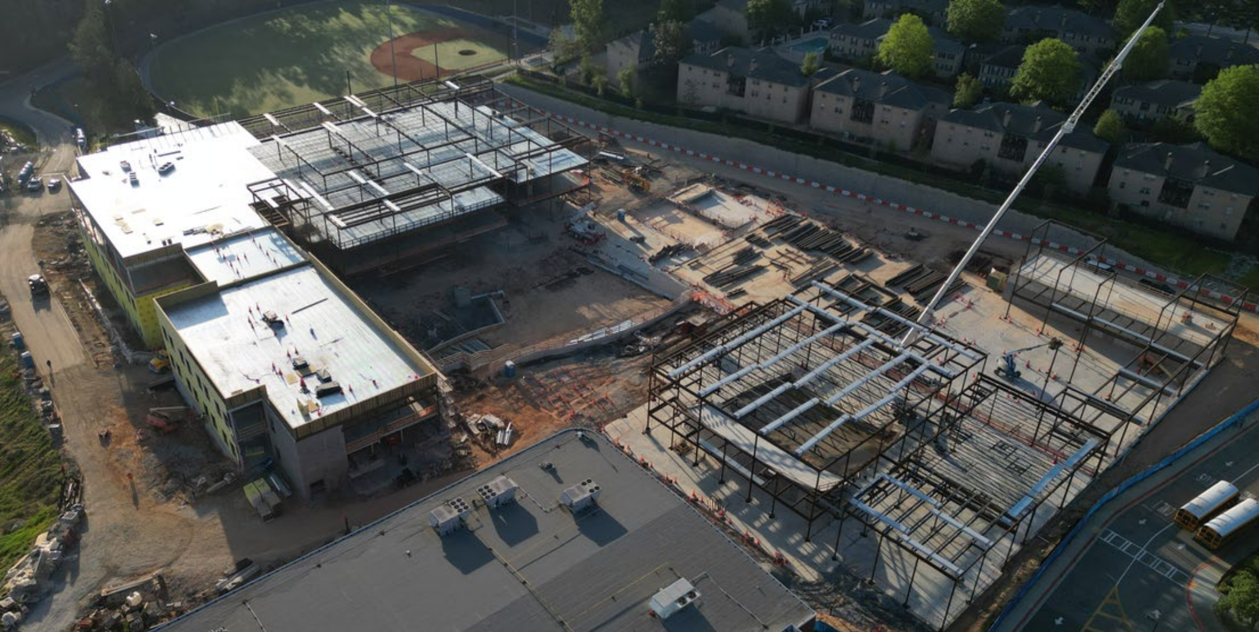
Overall Site Progress
