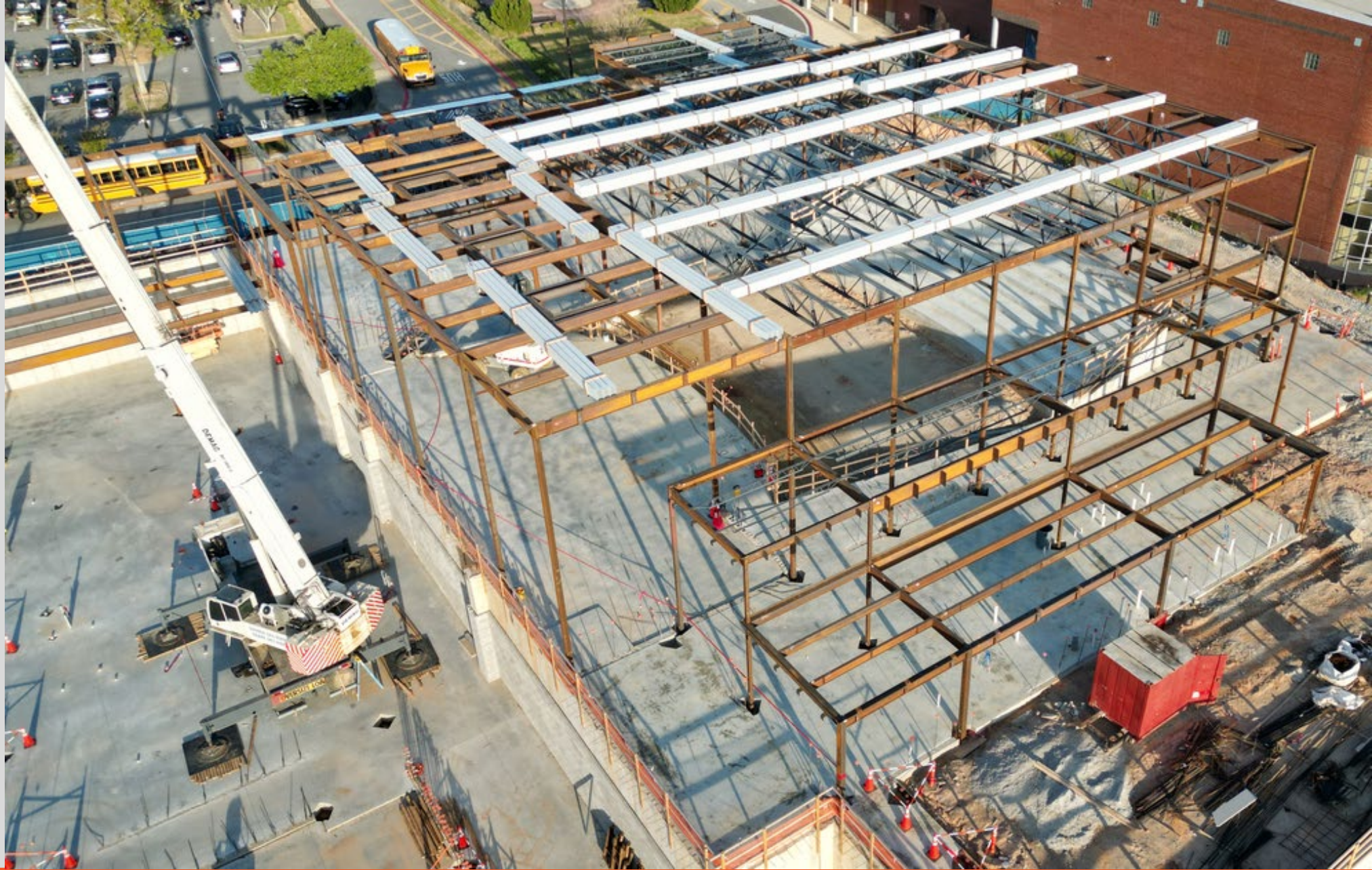
Auditorium – Area 8- Steel Erection and Roofing
