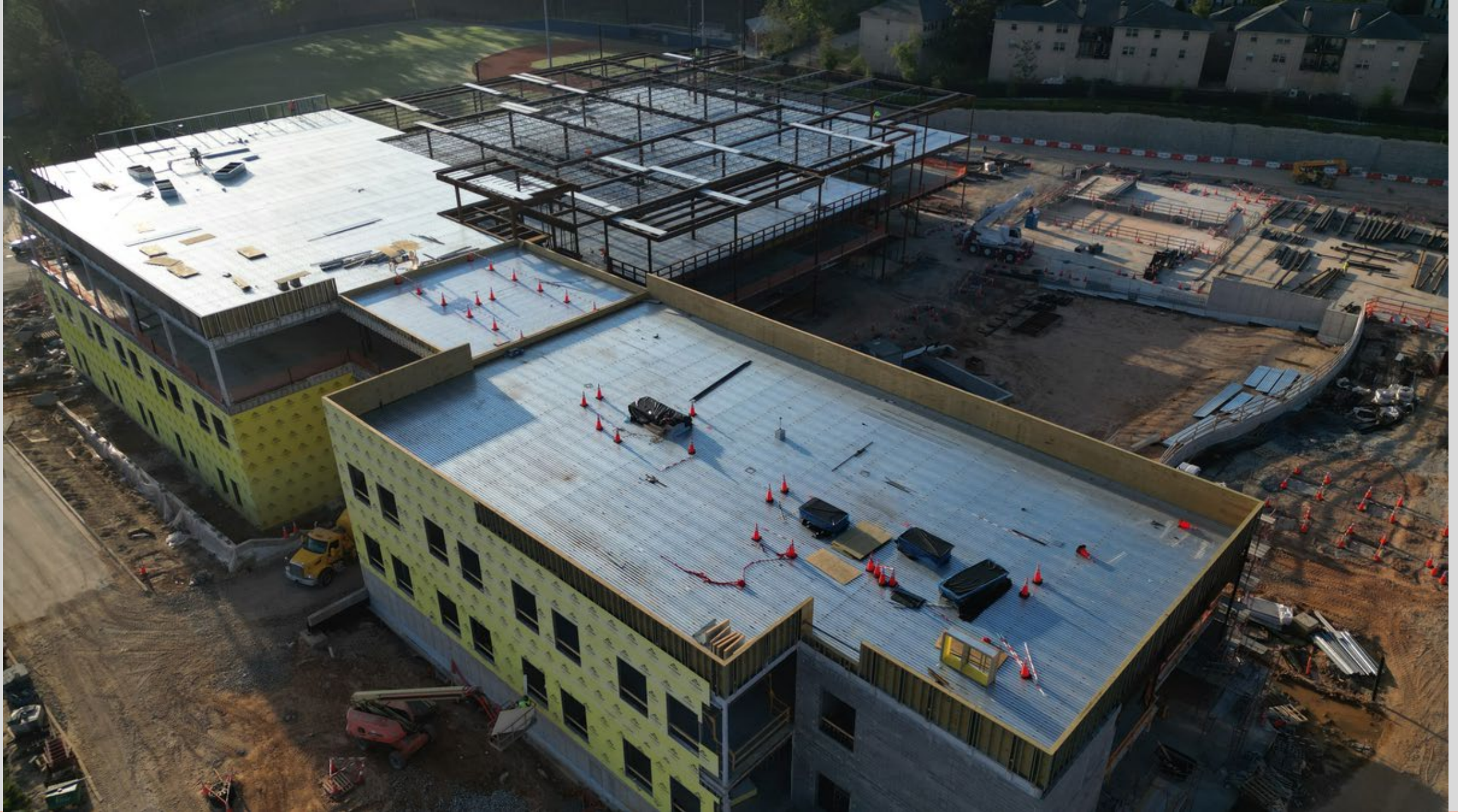
Area 2, 3 and 4 Roof.
