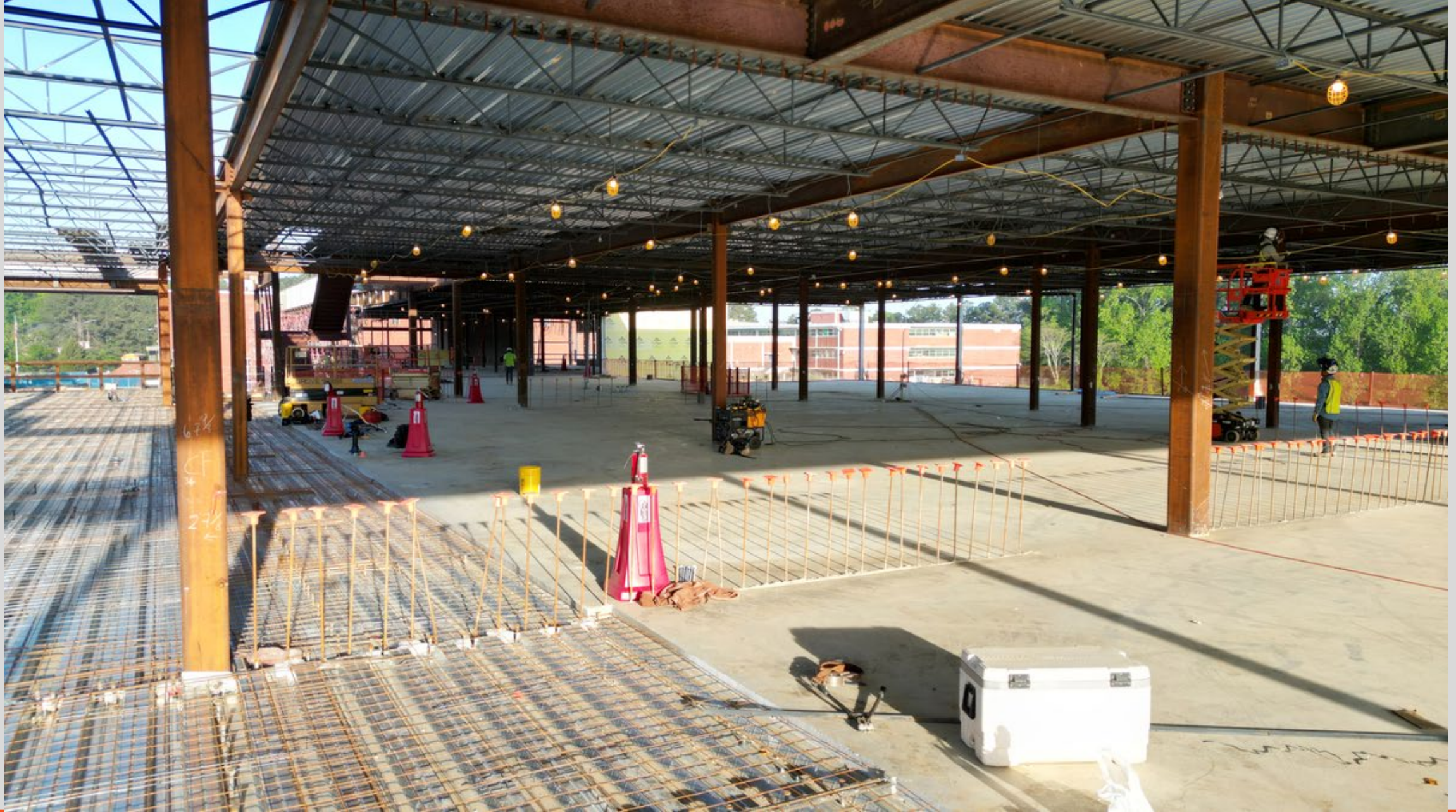
Area 4 LVL 3 Roof.
