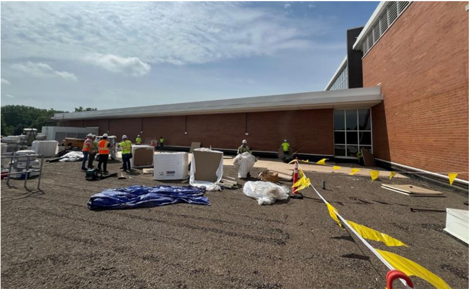
From top left: Area C re-roofing area above loading dock; closeup of roofing (July 2025)
