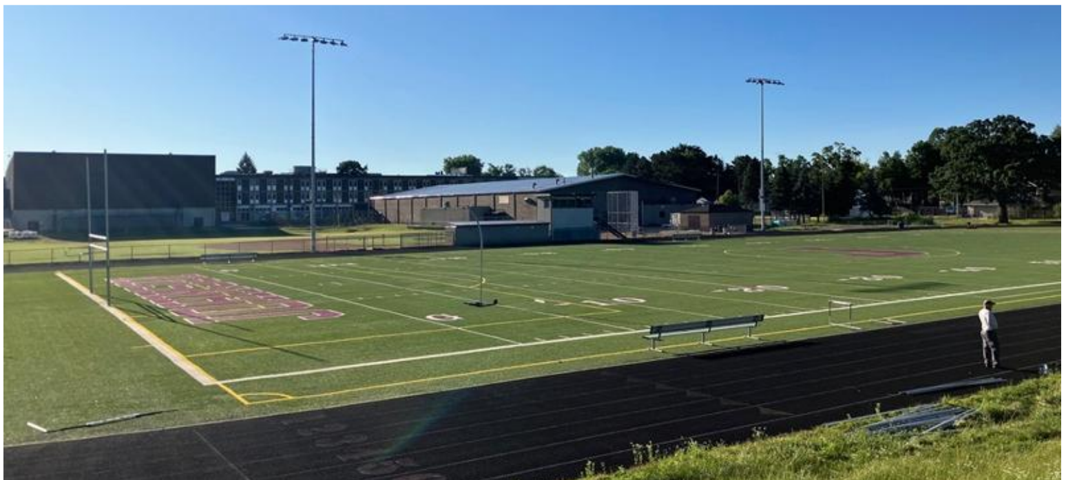
From top left: Bleacher footings being installed as seen in the background; bleacher footings in foreground; two poles with new field lighting (July 2025)
