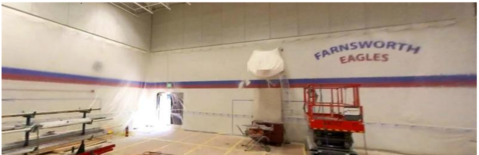
From top left: Classroom ceiling; lights and tile; classroom technology mockup; gym acoustic panel and paint (July 2025)
