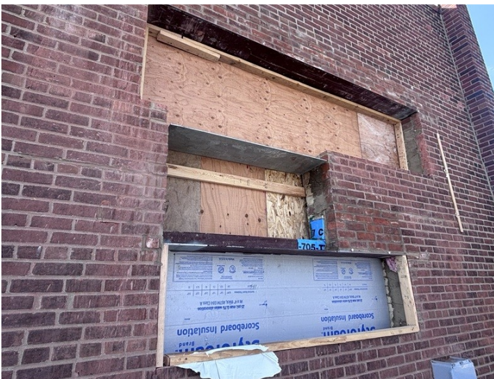
From top: New mechanical equipment in updated fourth-floor penthouse; preparing exterior wall for penthouse louvers; second-floor above-ceiling work (March 2026)
