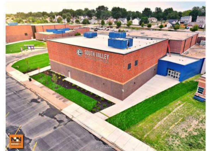
SVMS Exterior View
