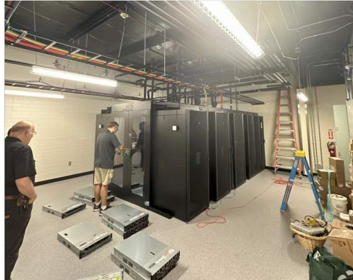
Data Pod Install
