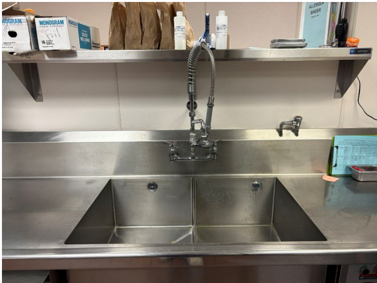
Kitchen South Tap – Sample 31126-SIS-03, Lead at 5.9 ppb Kitchen South Sprayer – Sample 31126-SIS-04
