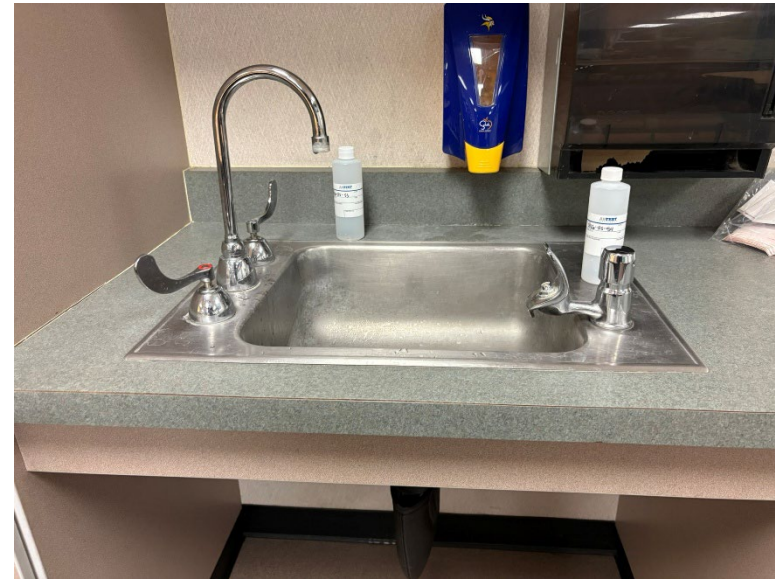
Room 316 Tap – Sample 31126-SIS-53 Room 316 Fountain – Sample 31126-SIS-54
