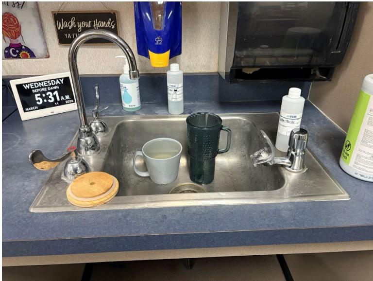
Room 209 Tap – Sample 31126-SIS-110 Room 209 Fountain – Sample 31126-SIS-111
