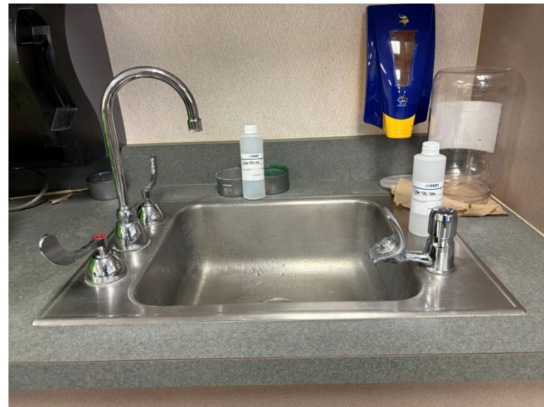
Room 310 Tap – Sample 31126-SIS-65 Room 310 Fountain – Sample 31126-SIS-66
