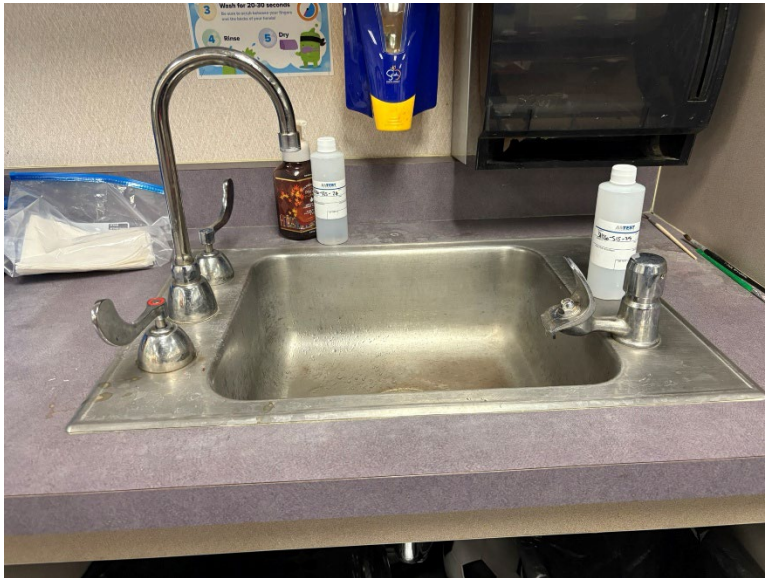
Room 103 Tap – Sample 31126-SIS-24 Room 103 Fountain – Sample 31126-SIS-25
