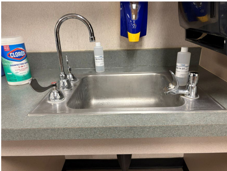
Room 309 Tap – Sample 31126-SIS-63 Room 309 Fountain – Sample 31126-SIS-64
