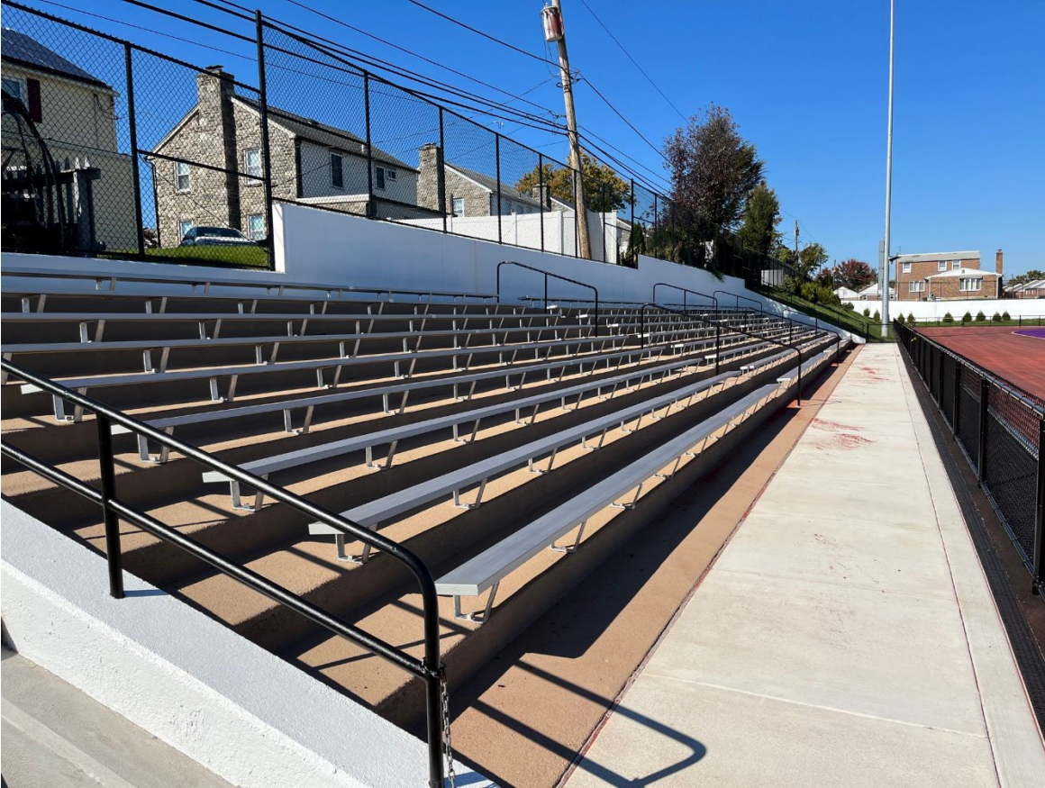
Rehabilitated Existing Concrete Home Bleacher
