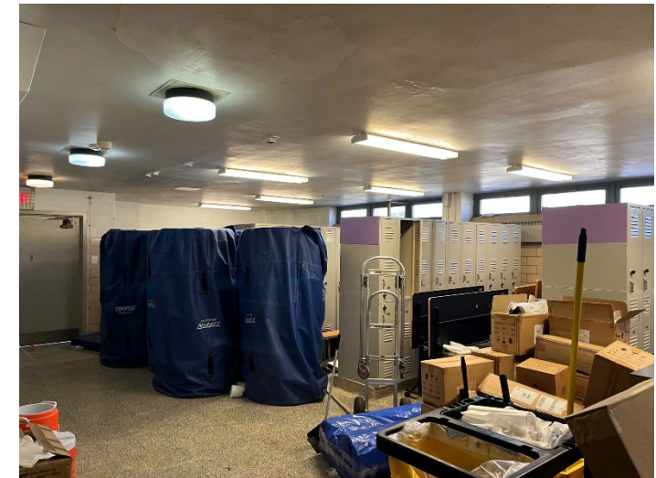
DH Locker Room Before Renovation
