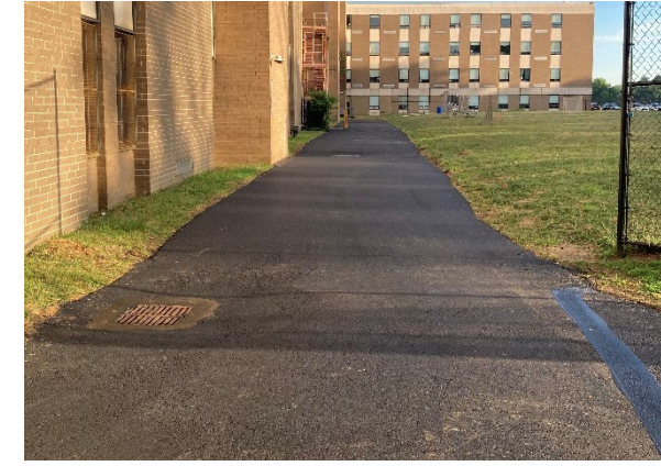
HS Paving – Around Practice Field
