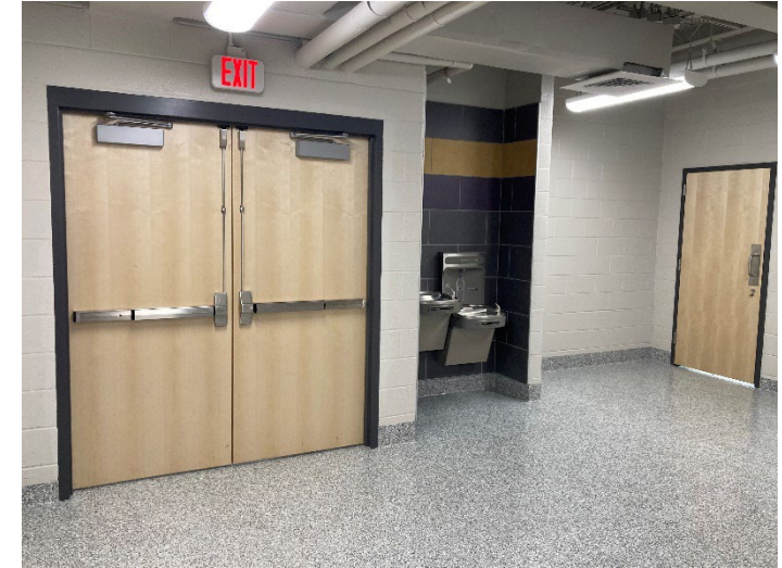
DH Locker Room After Renovation
