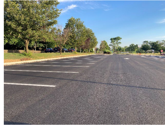
HS Parking Lot / Later Added Numbers
