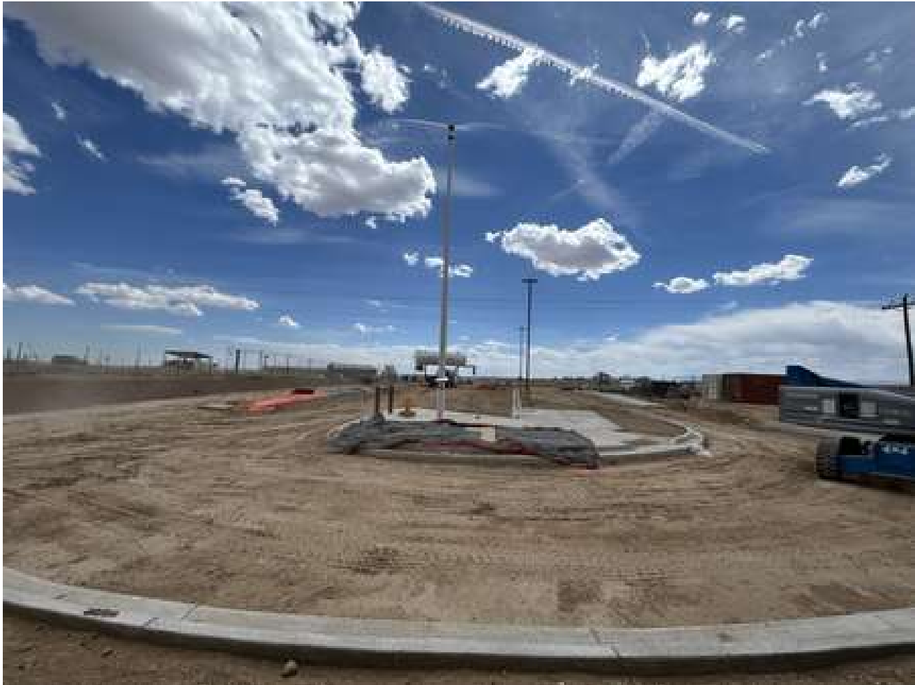
New Flagpole at Drop Off
