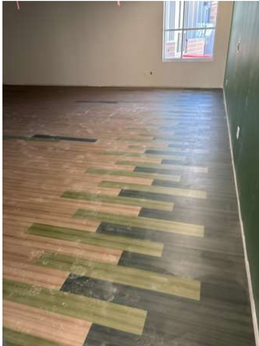
Floor in New Classroom
