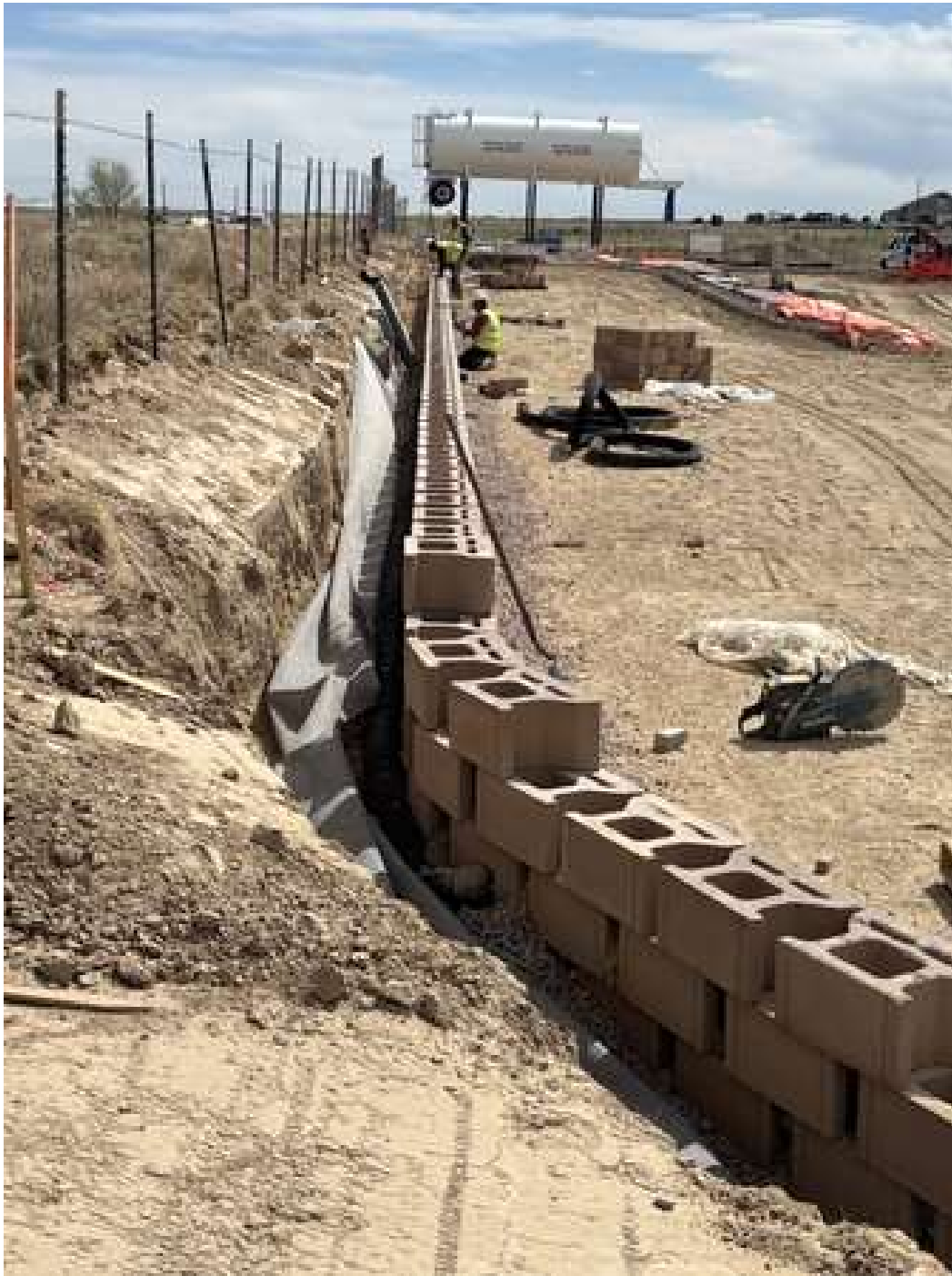
New Retaining Wall
