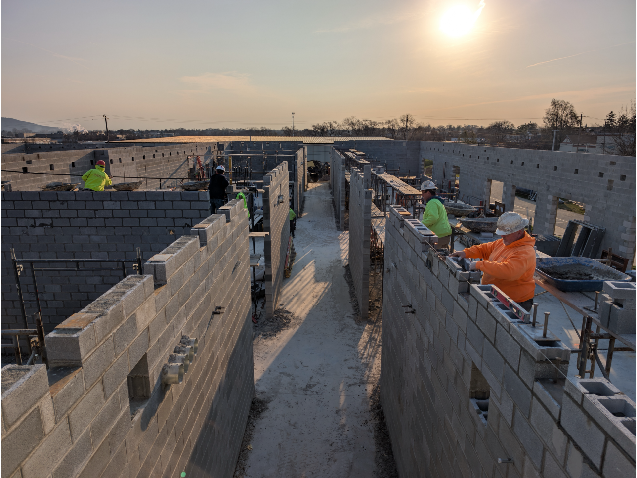
South Wing Area D Addition Progress
