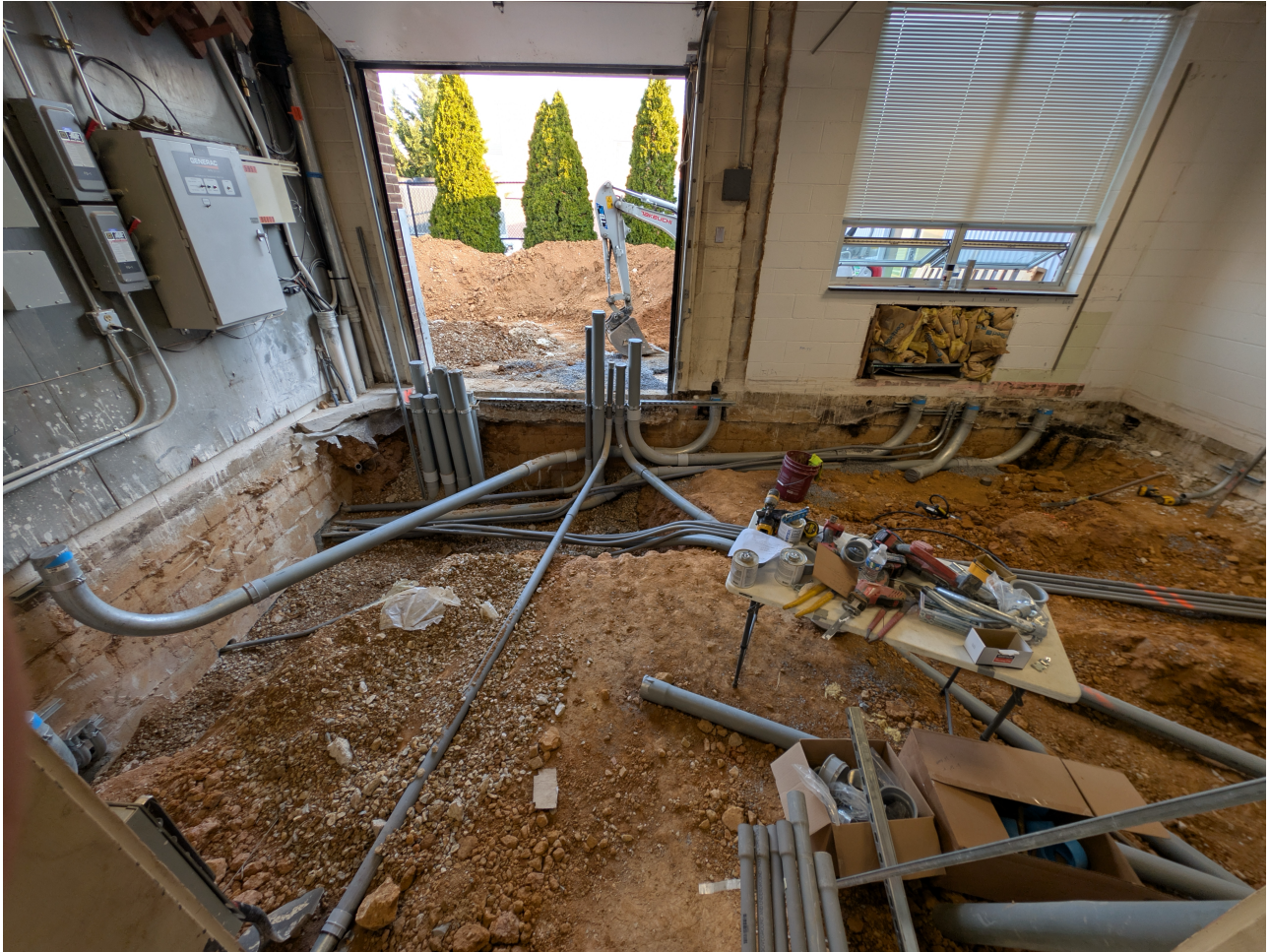
New Electric Room Underground Conduits
