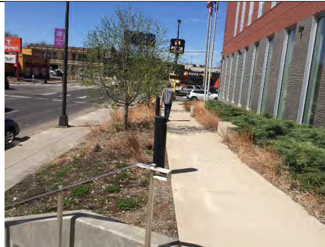
Stormwater planter after spring cleanup
