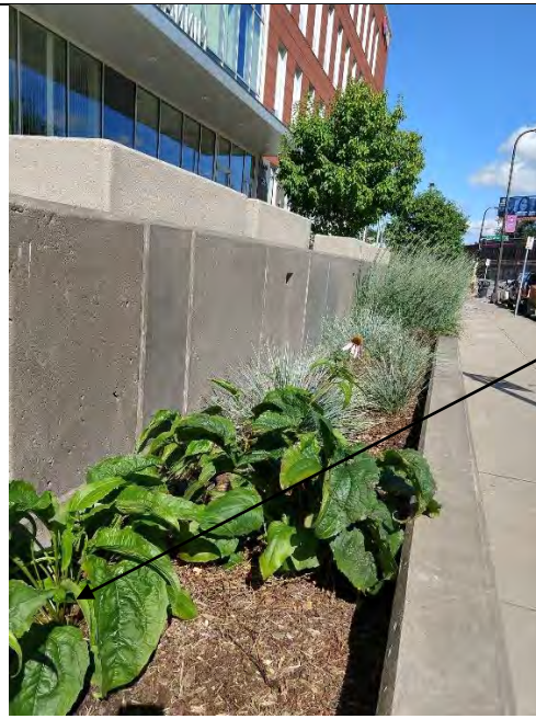
Stormwater planter on front of building captures sheetflow from sidewalk into landscaping beds
