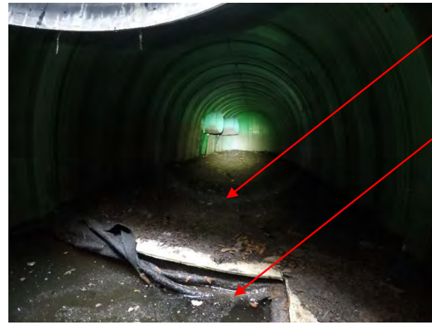
North Header row after final pass of jetter and vacuum
