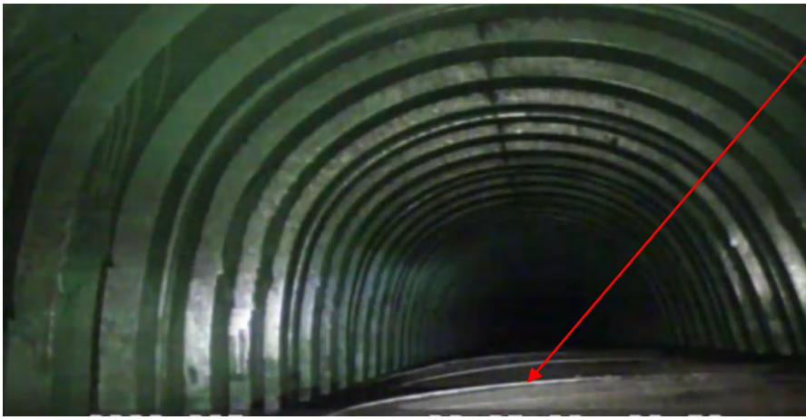
North Header row after final pass of jetter and vacuum
