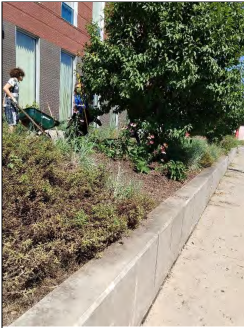
Stormwater planter on front of building captures sheetflow from sidewalk into landscaping beds
