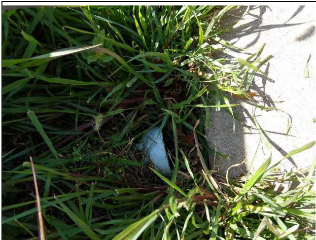
Underdrain outlet at west end of planter
