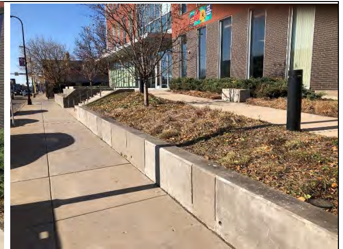
Stormwater planter after Fall cleanup
