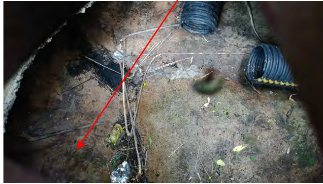
Under drains connecting to overflow
