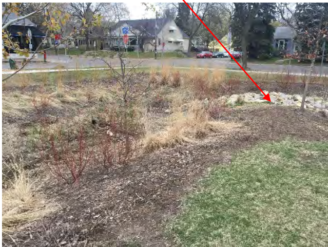
Overflow Structure from infiltration basin
