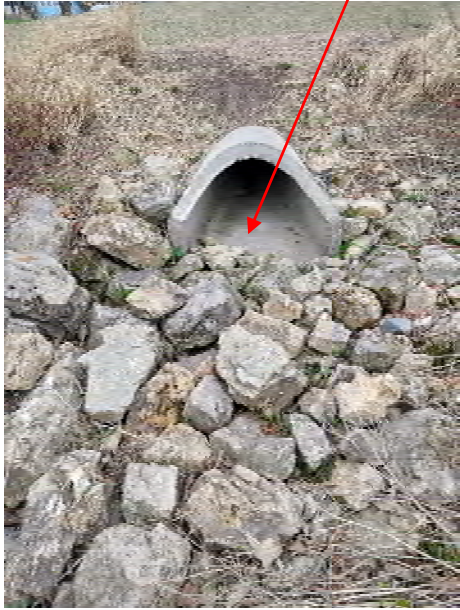
Inlet from roof of building
