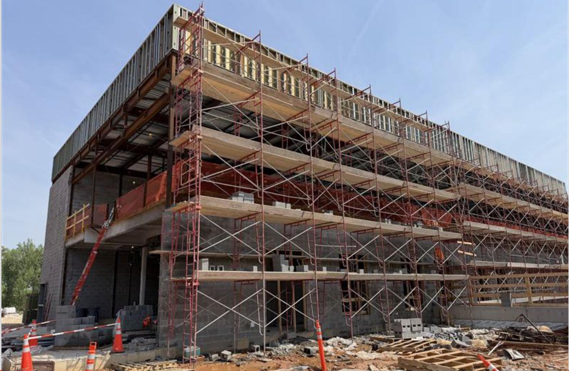
Exterior Framing and CMU work
