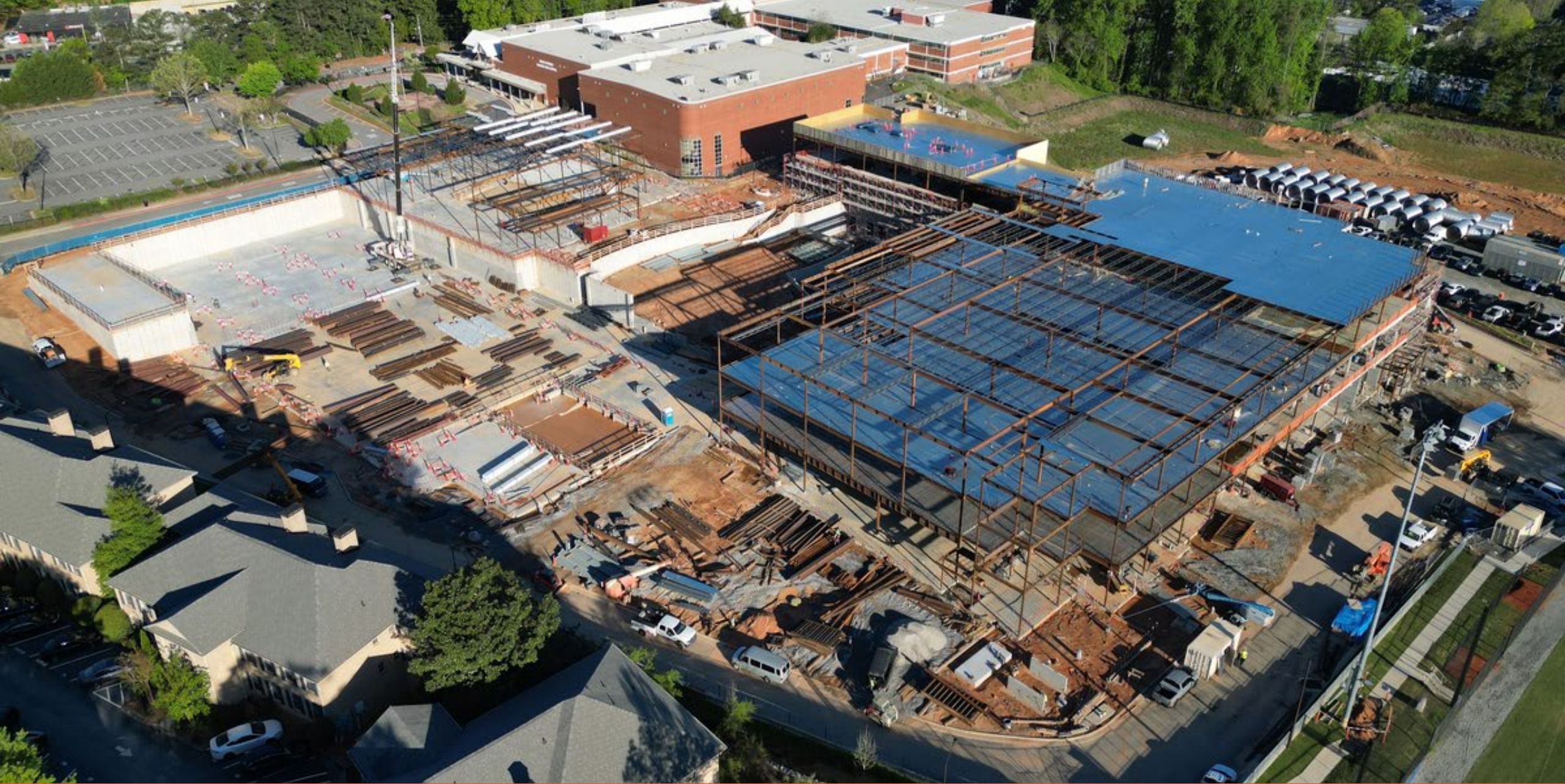
View from South-East- Roofing Work started
