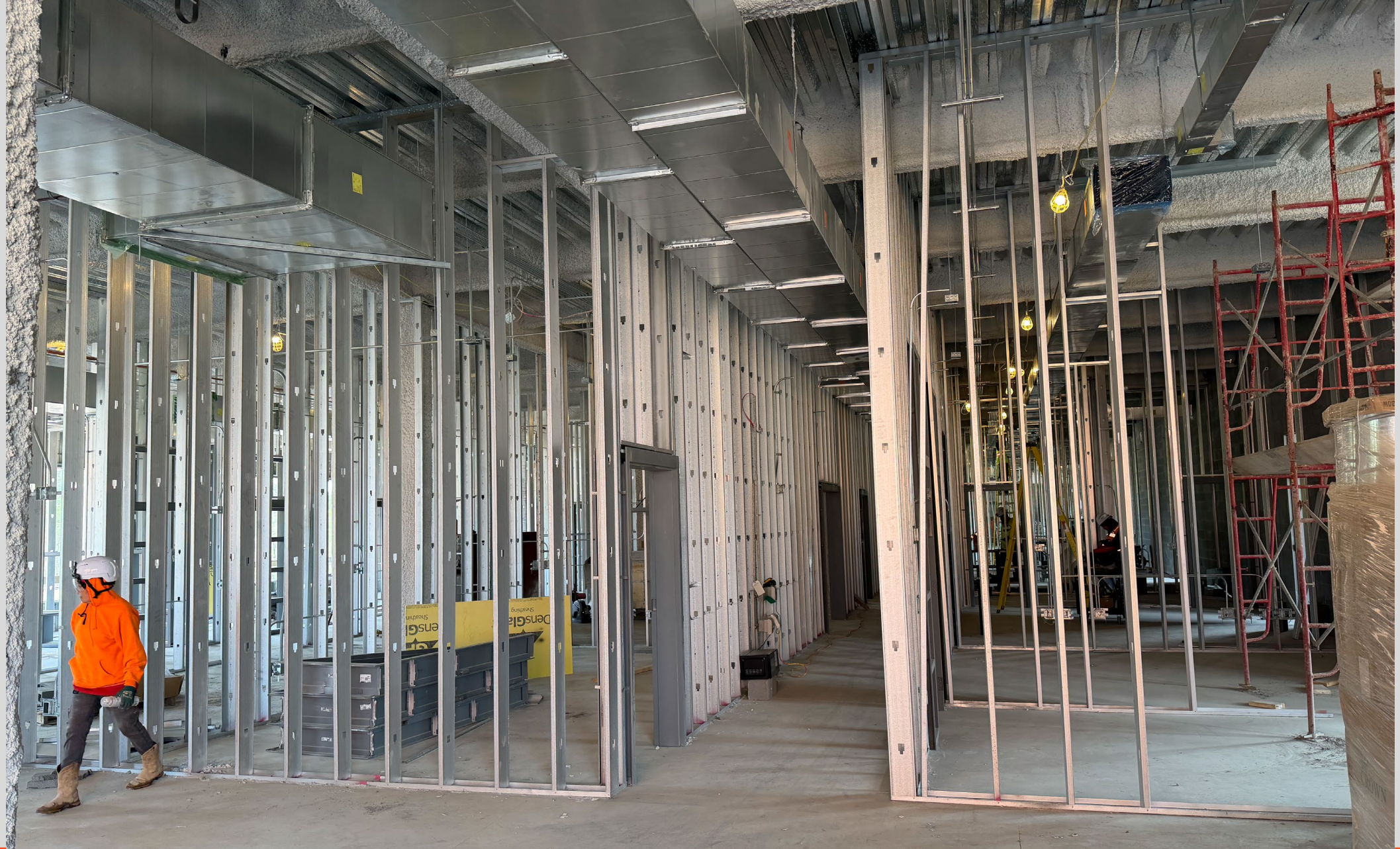
Interior Metal Framing work
