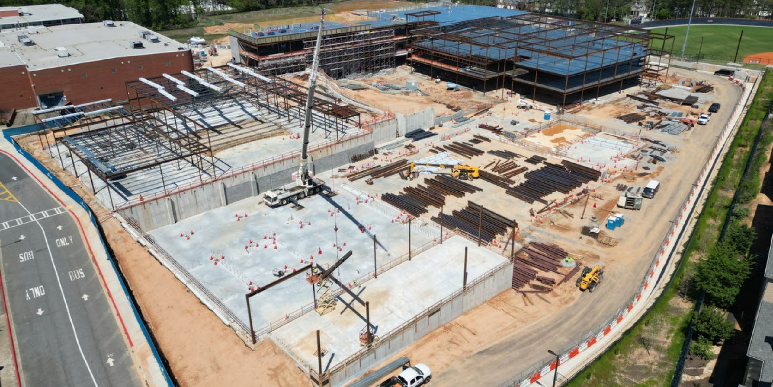
View from South-West- Area 8- Auditorium Steel Erection in Progress
