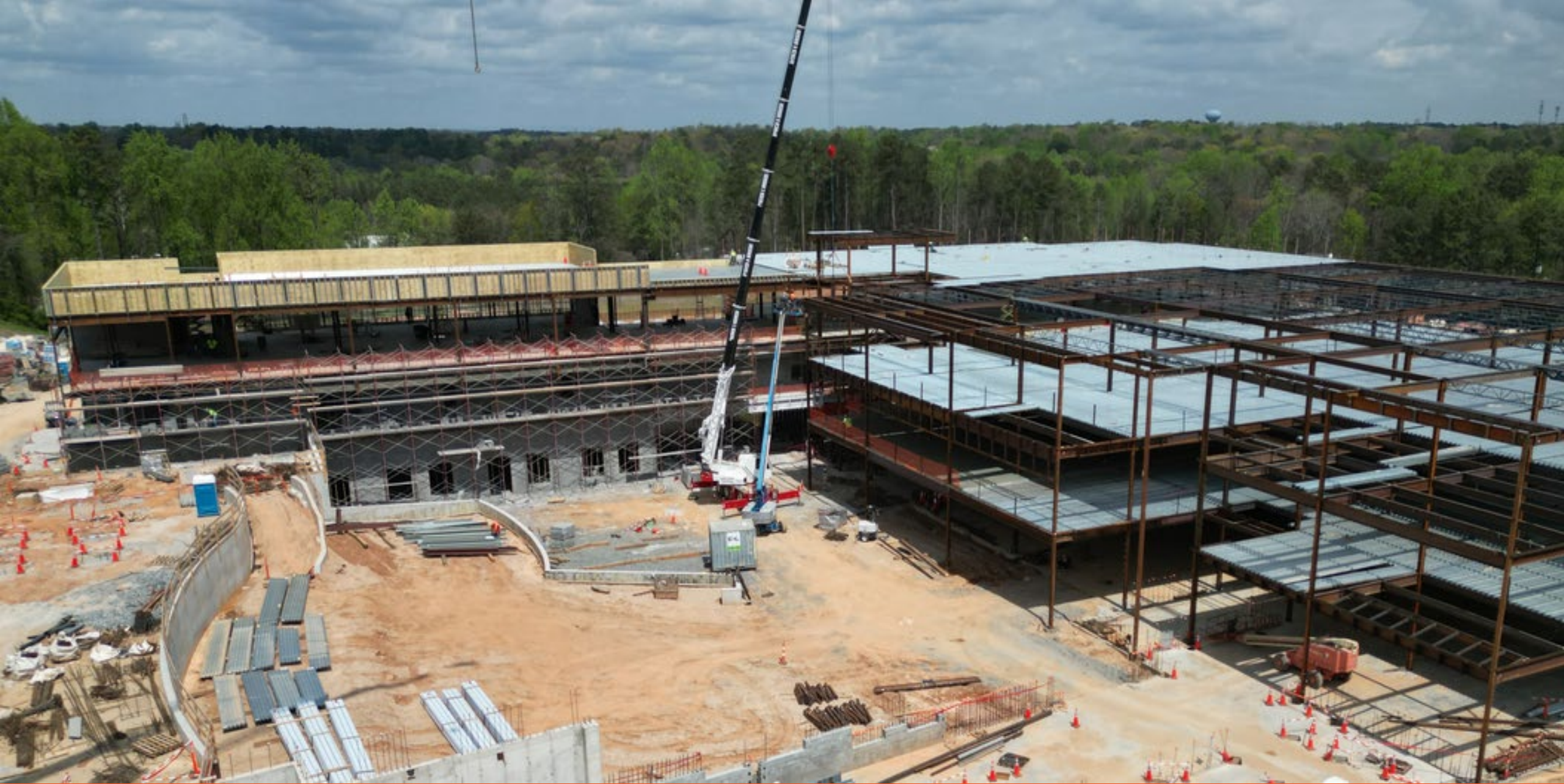
Exterior Framing and Interior CMU work
