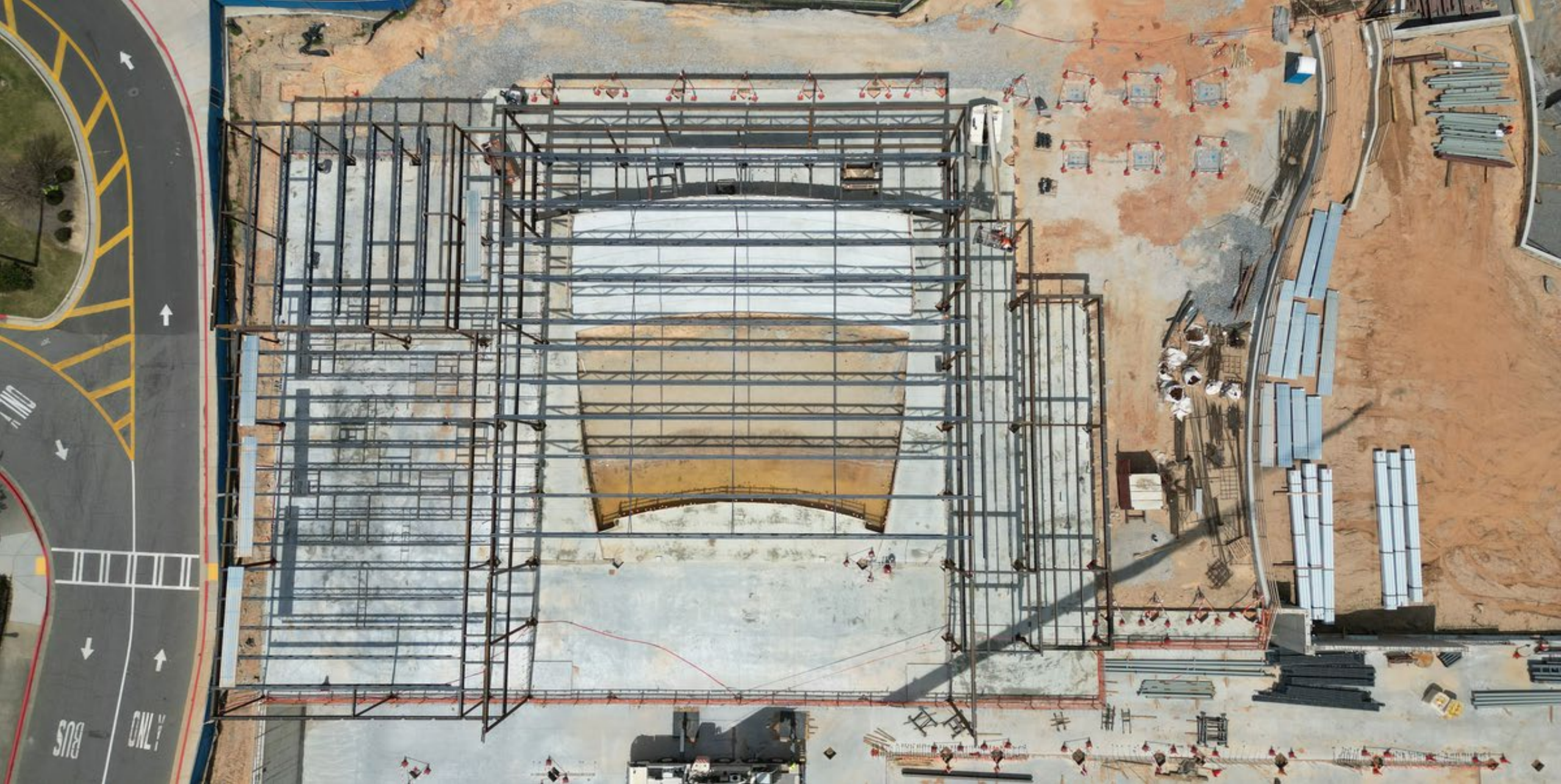
Area 8- Auditorium Steel Erection in Progress
