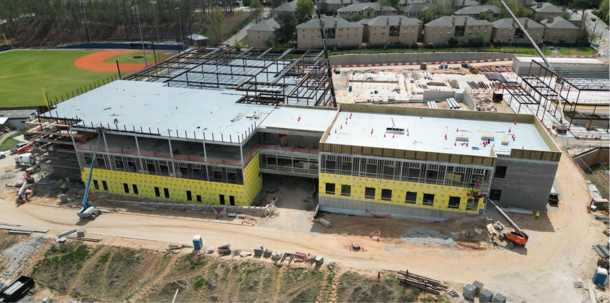
North Elevation- Exterior Framing and Steel Erection work
