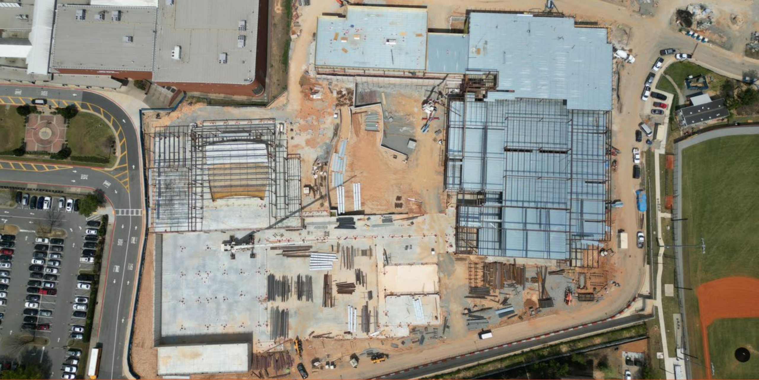
Overall Site Progress
