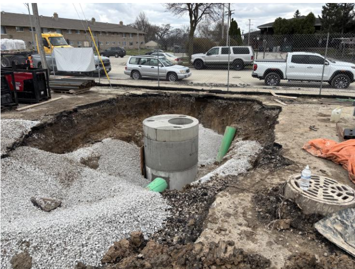
Storm Structure Install- South Entrance
