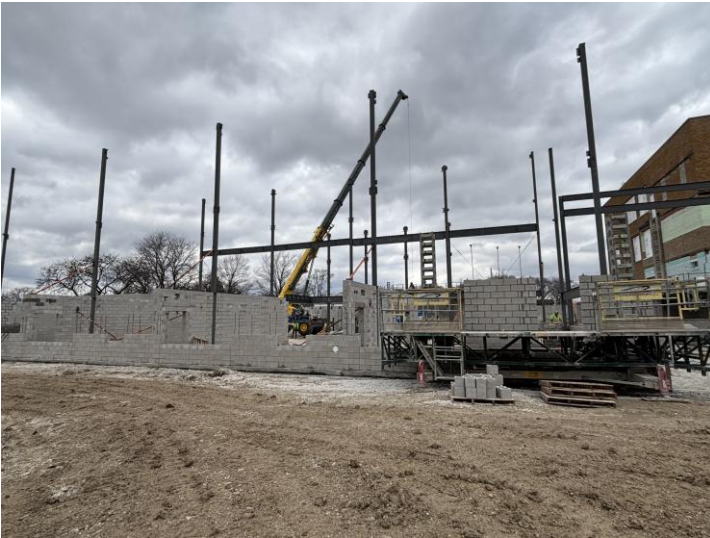
Structural Steel Erection- Vocational Training Rooms Area C
