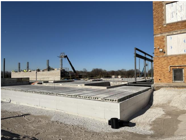
Precast Plank Completion & Additional Backfill Lift – Area B
