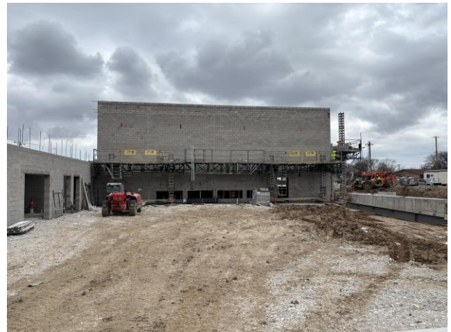
Masonry Top Out Of East Natatorium Wall – Area B
