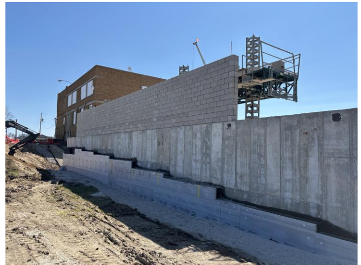
North CMU Wall - Gymnasium Building C
