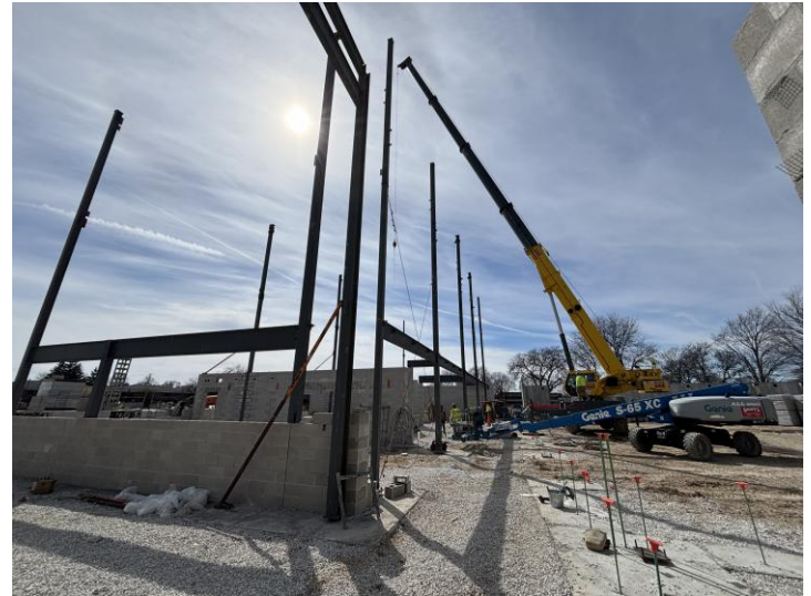
Structural Steel Erection- Main Entry Lobby & Corridor Area C
