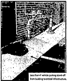
Main Gas Line Elementary Building
