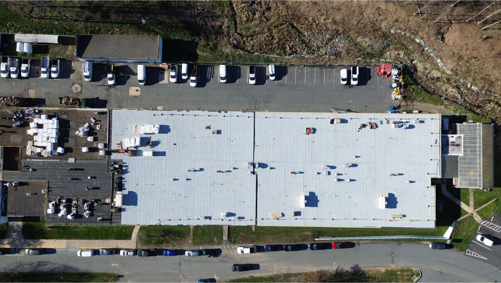
ADMINISTRATIVE SERVICES CENTER – ROOF REPLACEMENT
