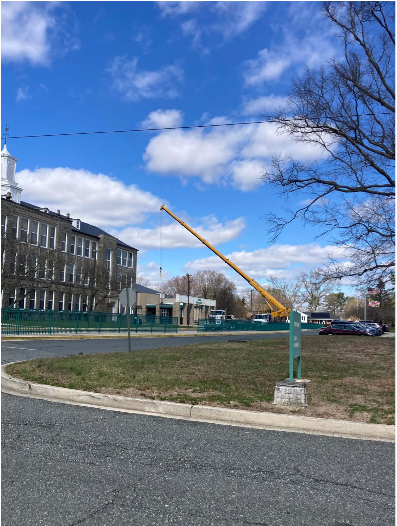
ELKTON MIDDLE SCHOOL - AC REPLACEMENT
