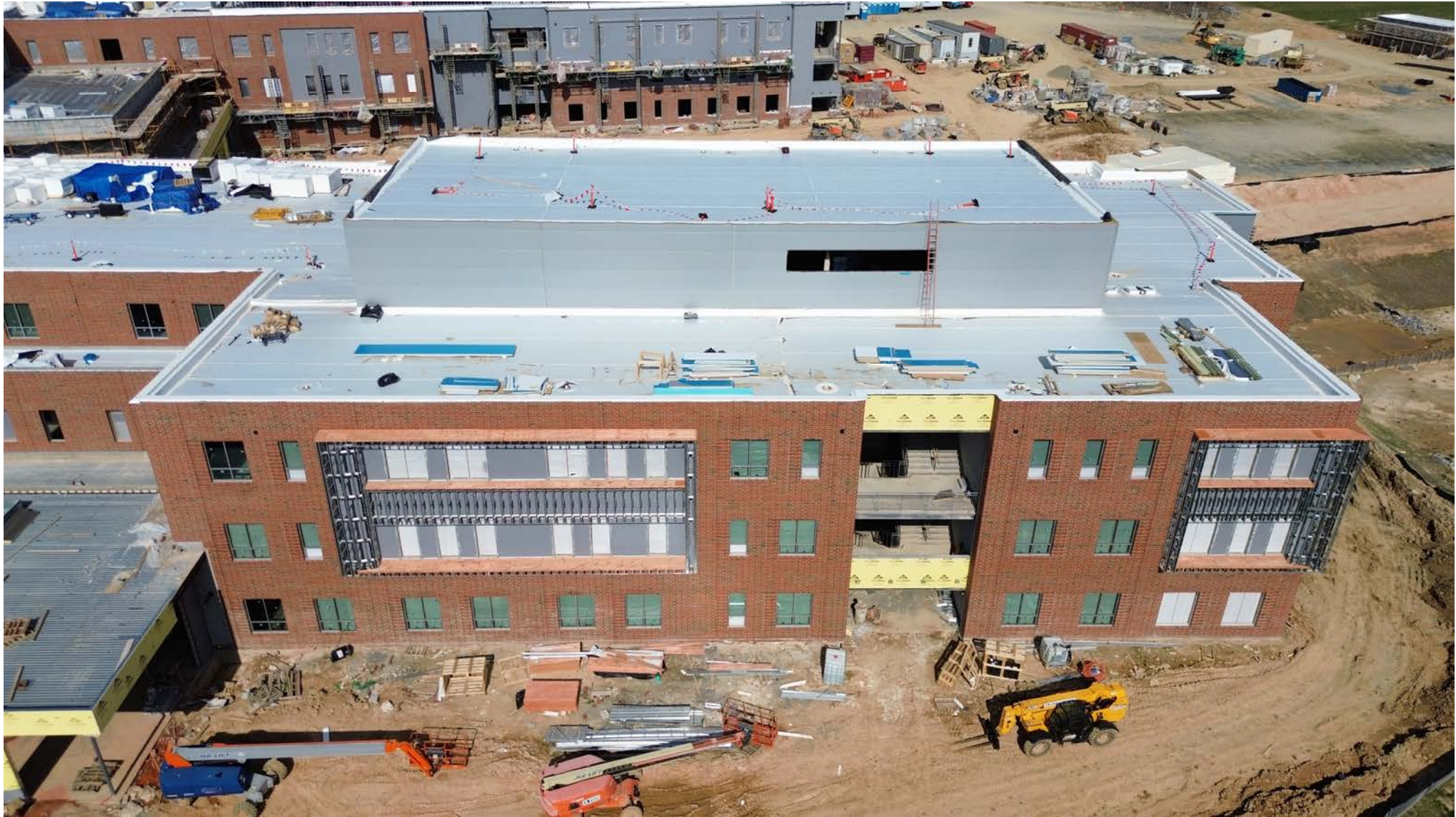
NORTH EAST MIDDLE / HIGH SCHOOL – REPLACEMENT – WINDOW INSTALLATION AND BRICK VENEER – MS WING
