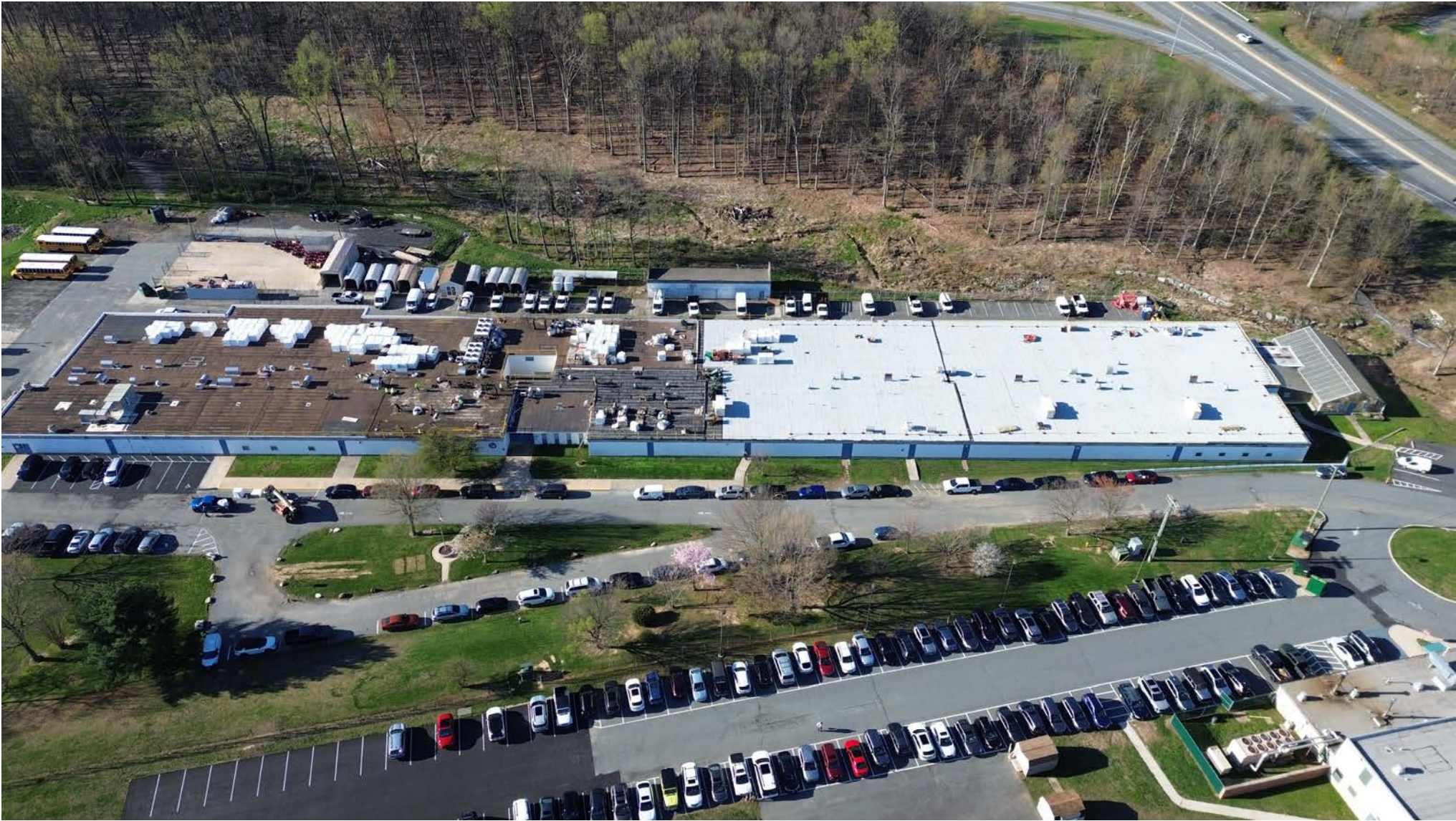
ADMINISTRATIVE SERVICES CENTER – ROOF REPLACEMENT
