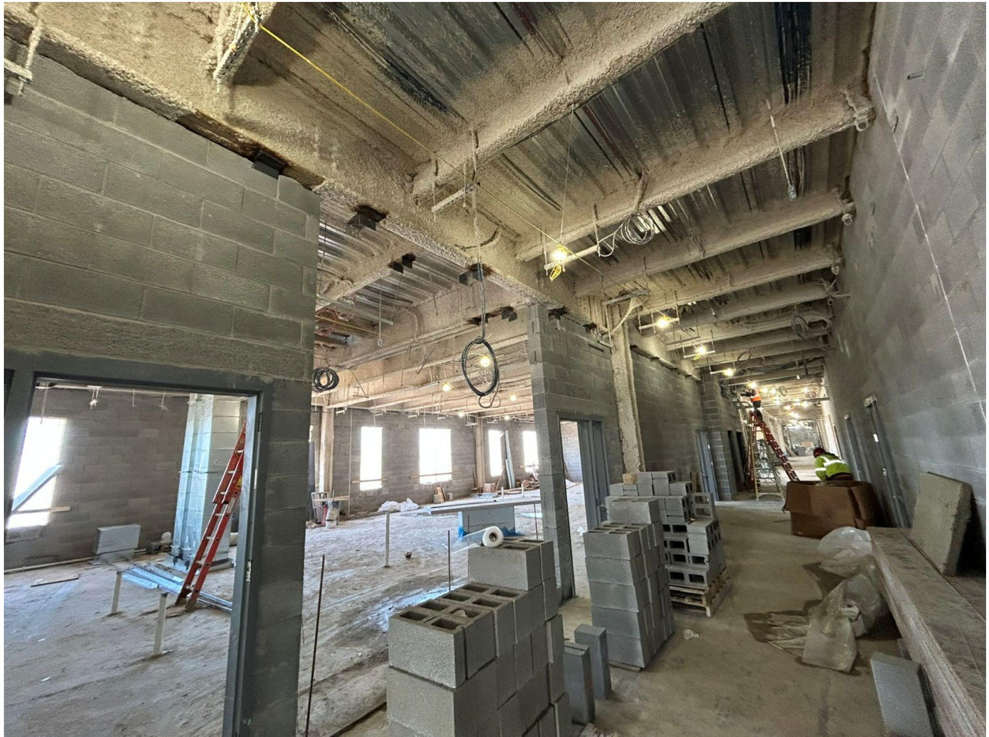
NORTH EAST MIDDLE / HIGH SCHOOL – REPLACEMENT – HS WING - FIREPROOFING
