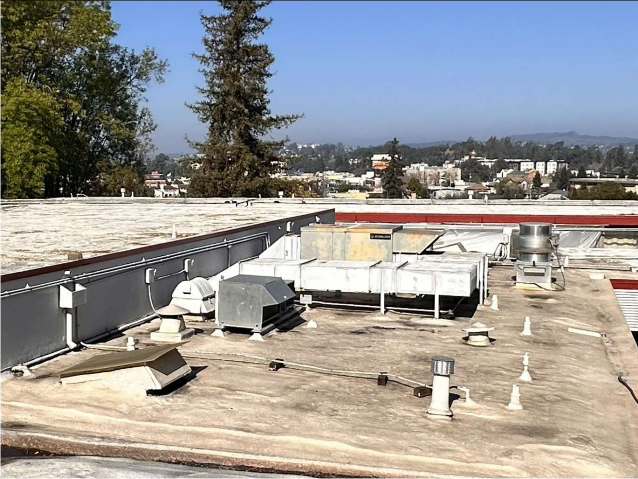
ROOF OUTSIDE EDGE
