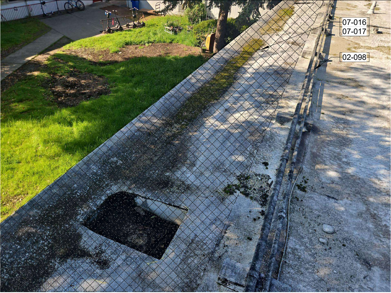
ROOF EDGE CONDITION
