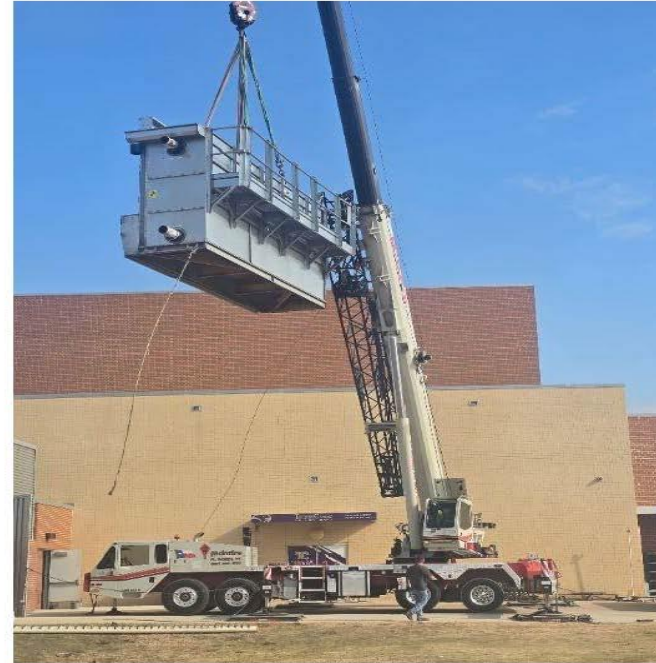
Crane positioning new coil assembly
