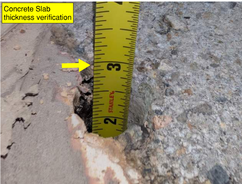
Total depth inspected for an under-slab vapor retarder
